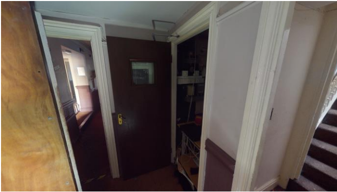
Photograph 12) Door to be removed and new partition installed
