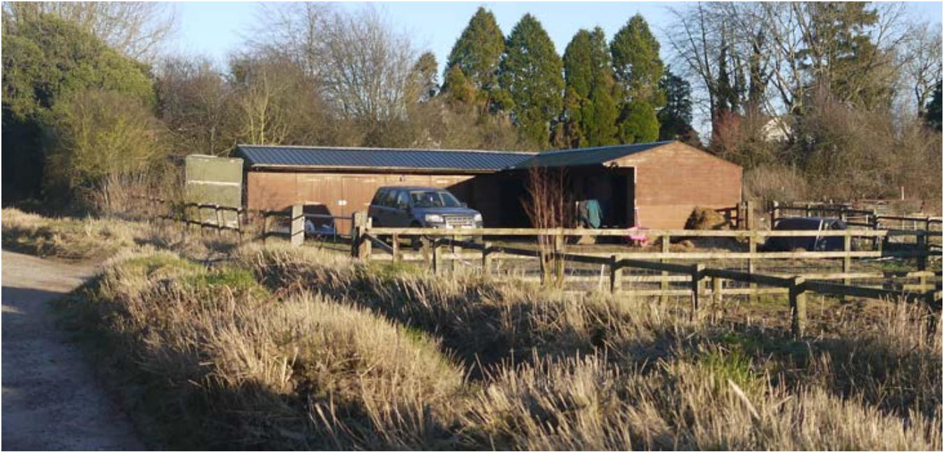
Example of stable block on Holmstead Road
