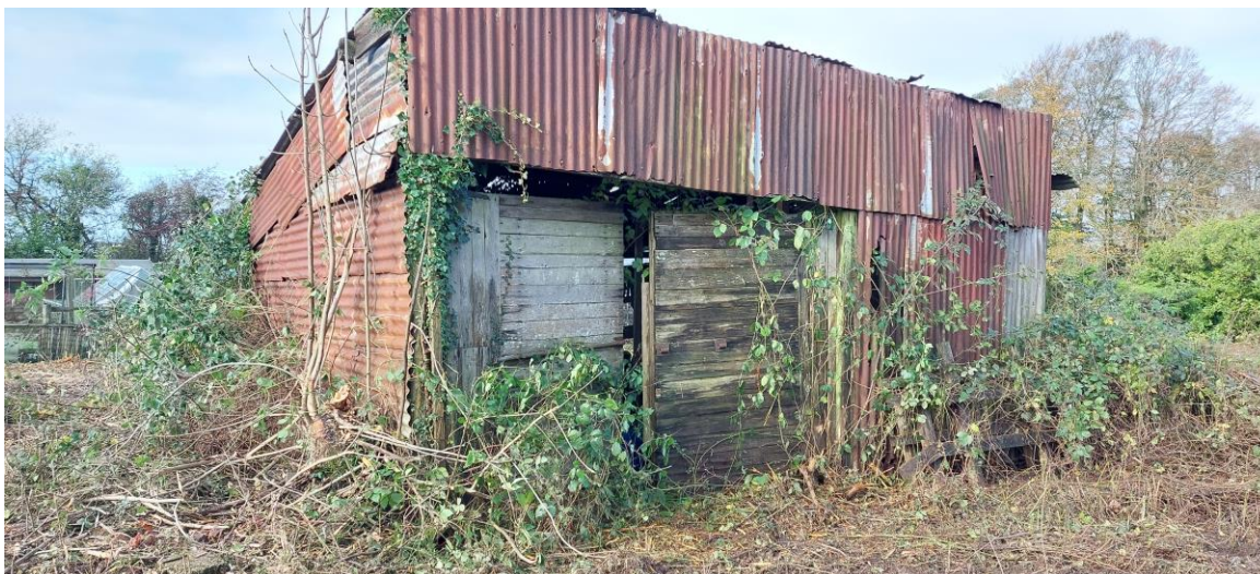
Image 07 – View of building B1 and scrub vegetation.
