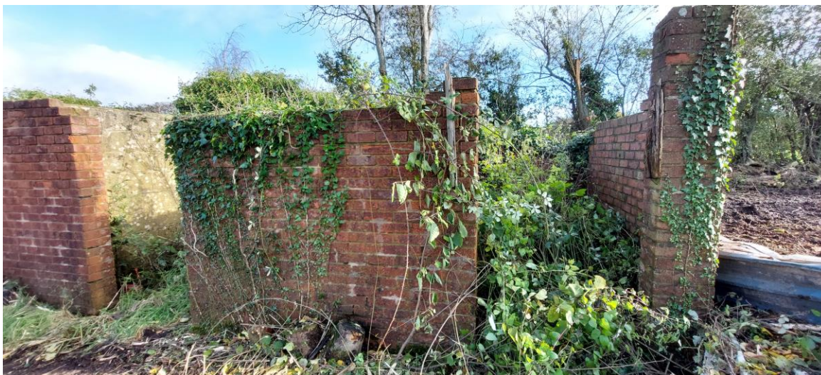
Image 08 – View of building B2 and scrub vegetation.
