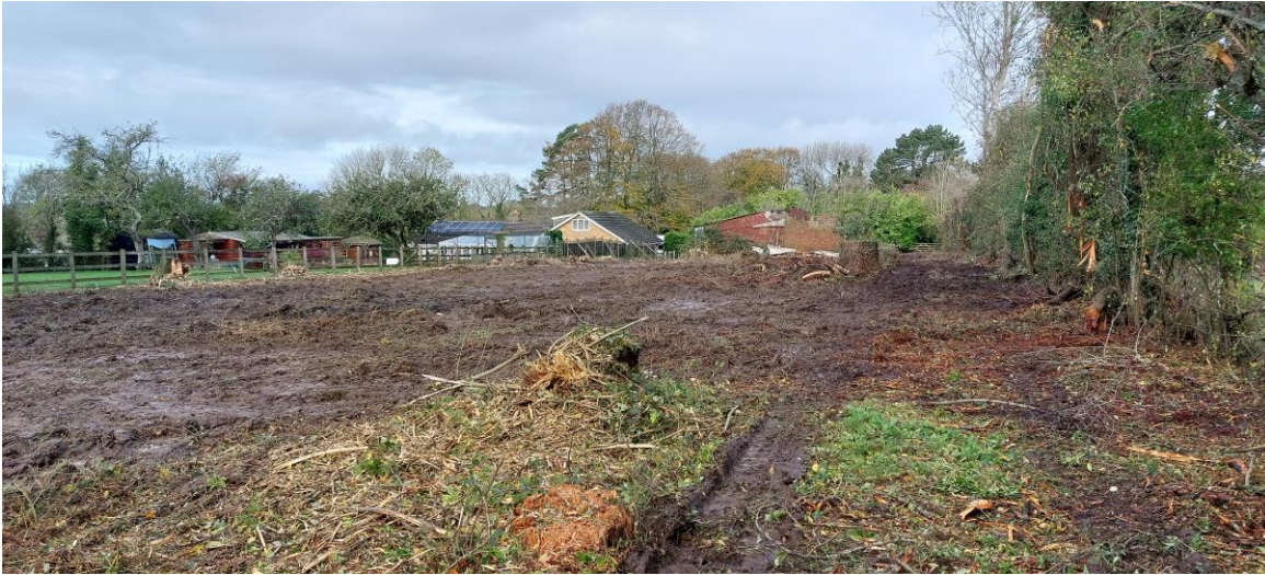
Image 03 – View of the site from south to north.
