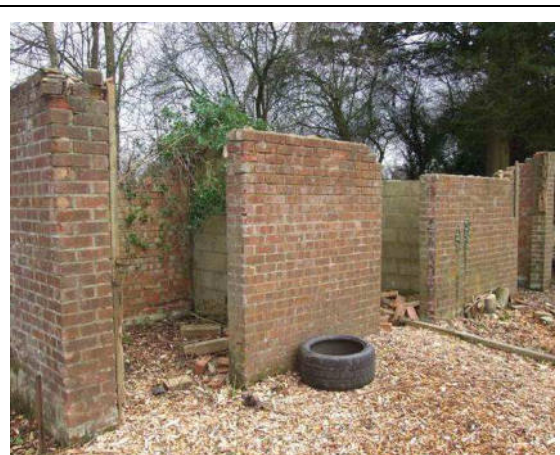
Photograph 4. Building B - brick outbuilding.
