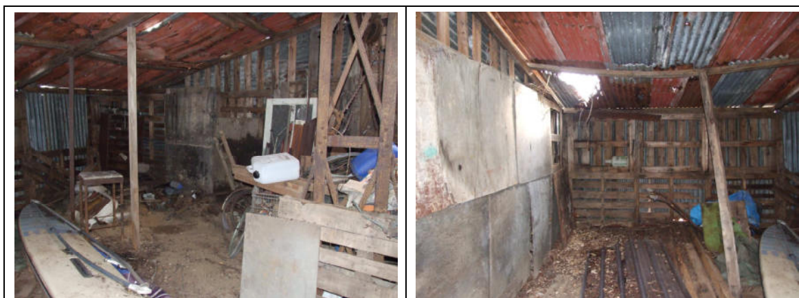
Photographs 6 and 7. Interior of building A.
