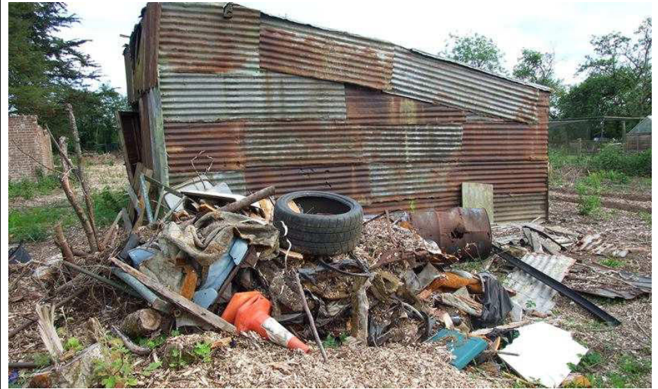
Photograph 13. Northern elevation of Building A and adjacent debris pile.
