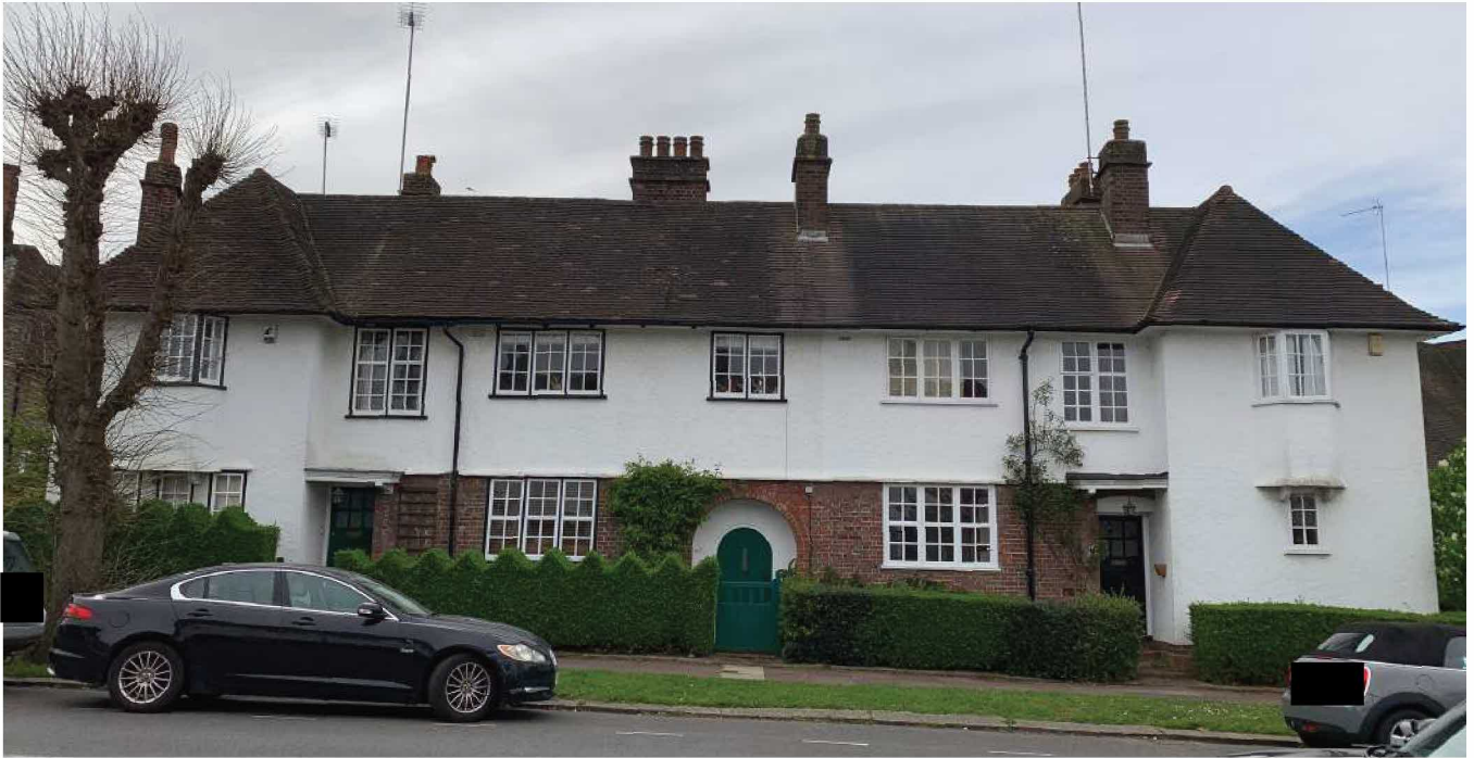
View to number 46 Temple Fortune Hill ( right ) showing the shared centre archway and adjoining house at number 48 ( left ).
