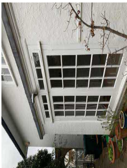
Top: View to the rear elevation; Bottom left: View to the existing outshot French doors. The doors are fixed shut and badly decayed and it is proposed that these are entirely replaced to match existing; Bottom right: View to the rear elevations to the adjoining houses at numbers 48 and 50.
