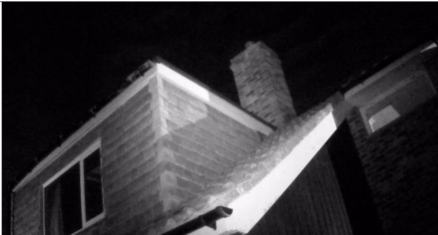
The 11 soprano pipistrelle emergences from the south-facing dormer detailed by surveyor 2 were also recorded by IR 2.
