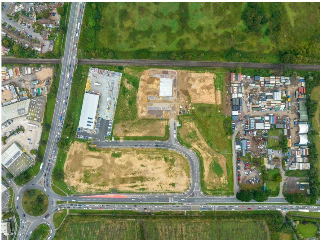
Aerial photograph of the wider development site (September 2023)
