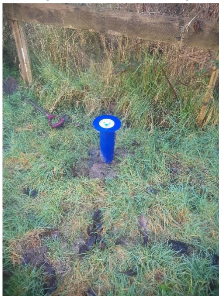
Fig 3. Groundwater monitoring well
