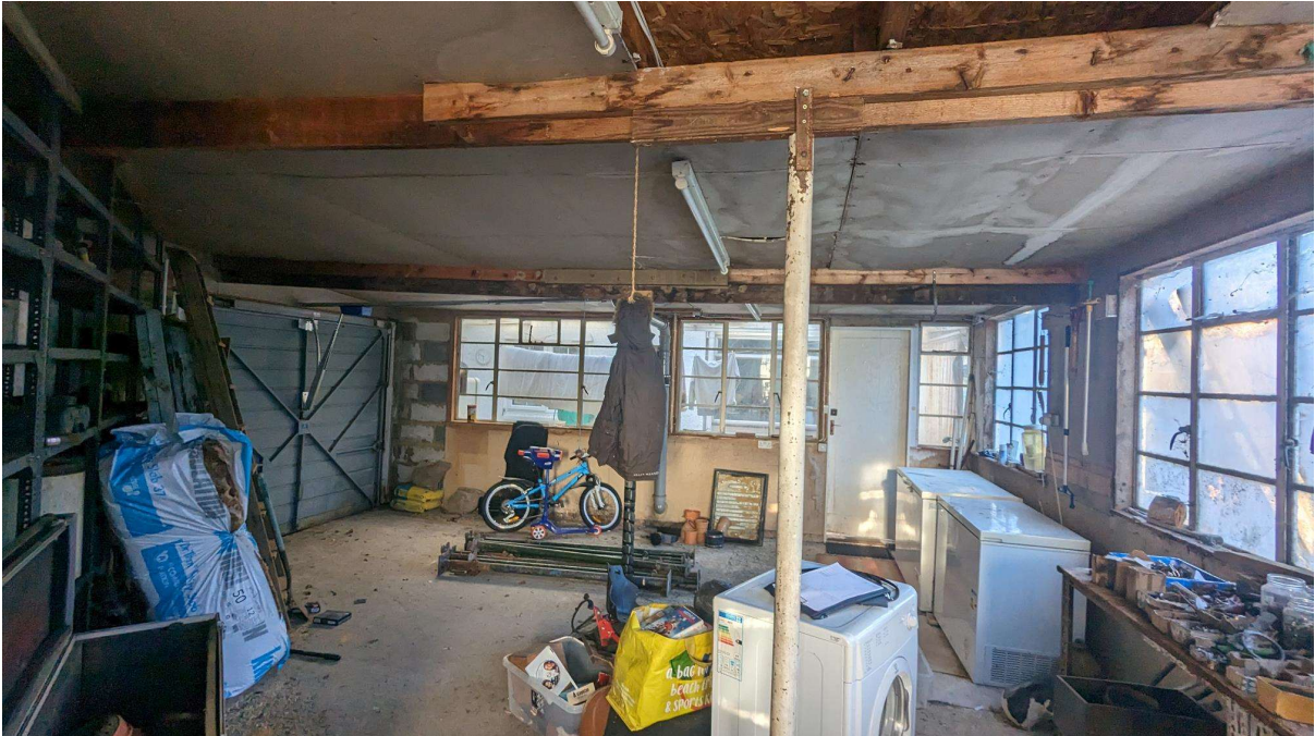
Photo 4 – View inside B2.
