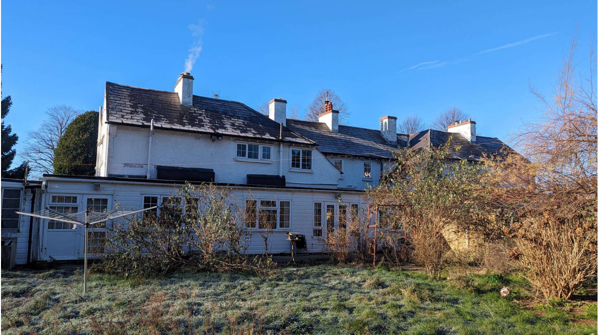
Photo 1 – View of the dwelling from the rear (east).
