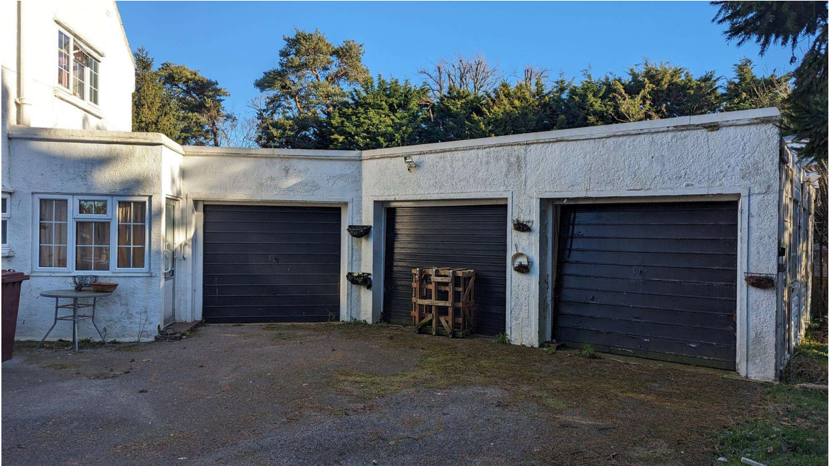
Photo 3 – View of the garage from the front (west).
