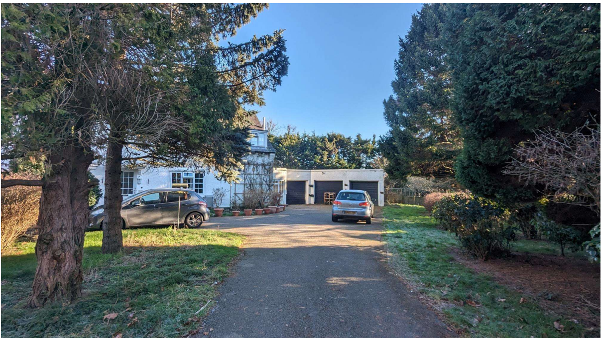
Photo 10 – View of the front driveway as you enter site.
