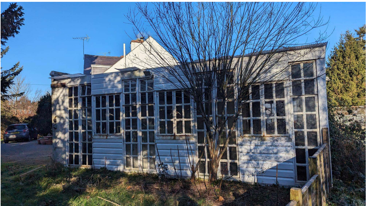
Photo 2 – View of the garage and store from the south.
