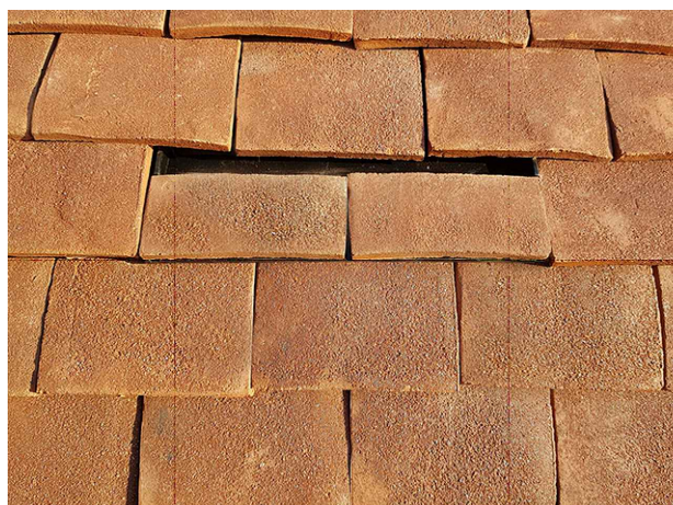
Proposed In line tile ventilator - Photo NTS
