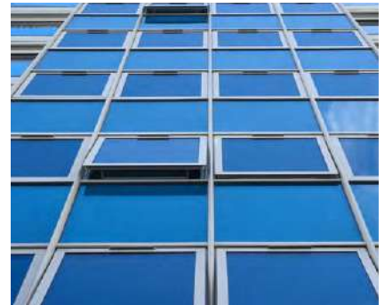
Aluminium clad curtain walling
