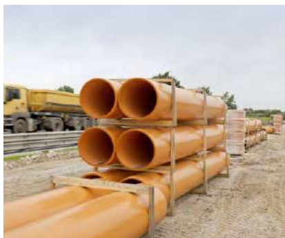
Polypropylene sewer pipe & chambers
