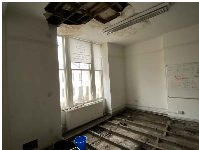
F001 - First Floor Front Office
