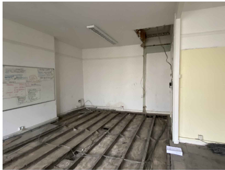
F001 - First Floor Front Office
