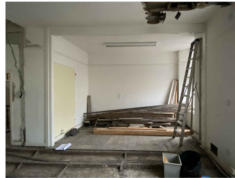
F001 - First Floor Front Office
