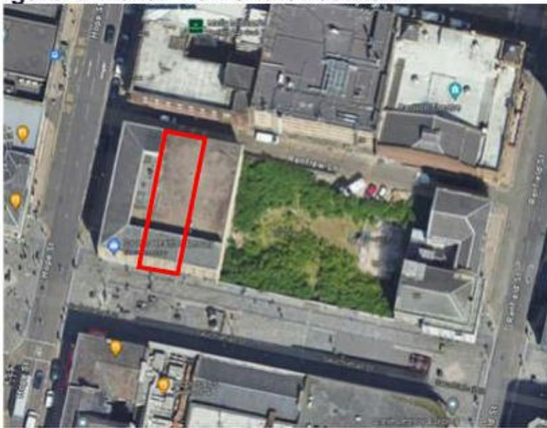
Figure 1. Aerial View and Streetview
