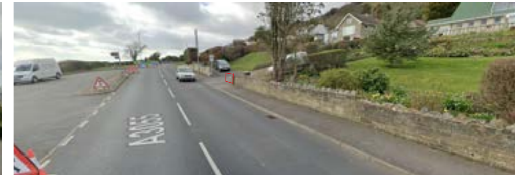
Fig 8 Approaching 71 Leeson Road from the East on Leeson Road (entrance outlined in red)
