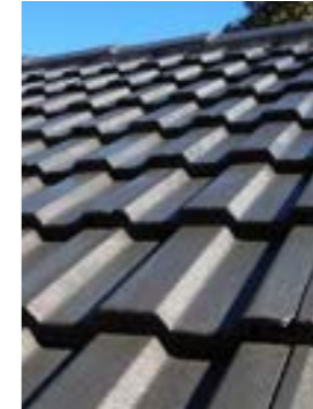
Existing concrete roof tiles to be painted black.
