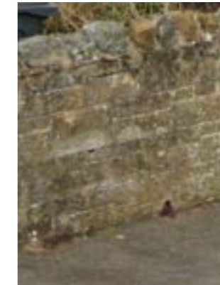
Ashlar brick & stone retaining front wall.
