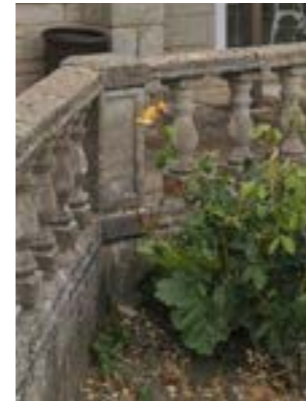
Concrete retaining wall/ balustrade
