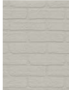
Light painted brickwork
