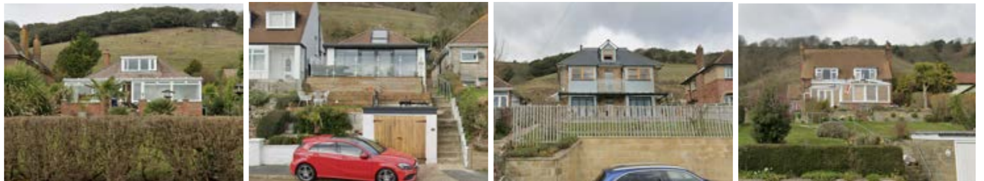
Fig 2 Properties along Leeson Road which have extended their houses to maximise on the views to the solent with the addition of glazing and extensions
