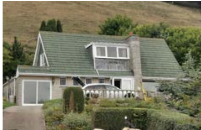
Fig 1 71 Leeson Road - South elevation
