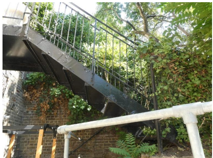
(Figure 3: Staircase side and lower view)
