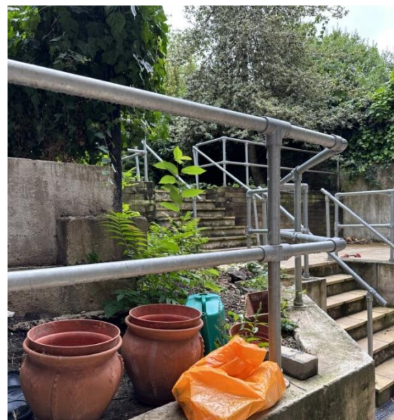
(Figure 5: Existing sets of steps in garden)
