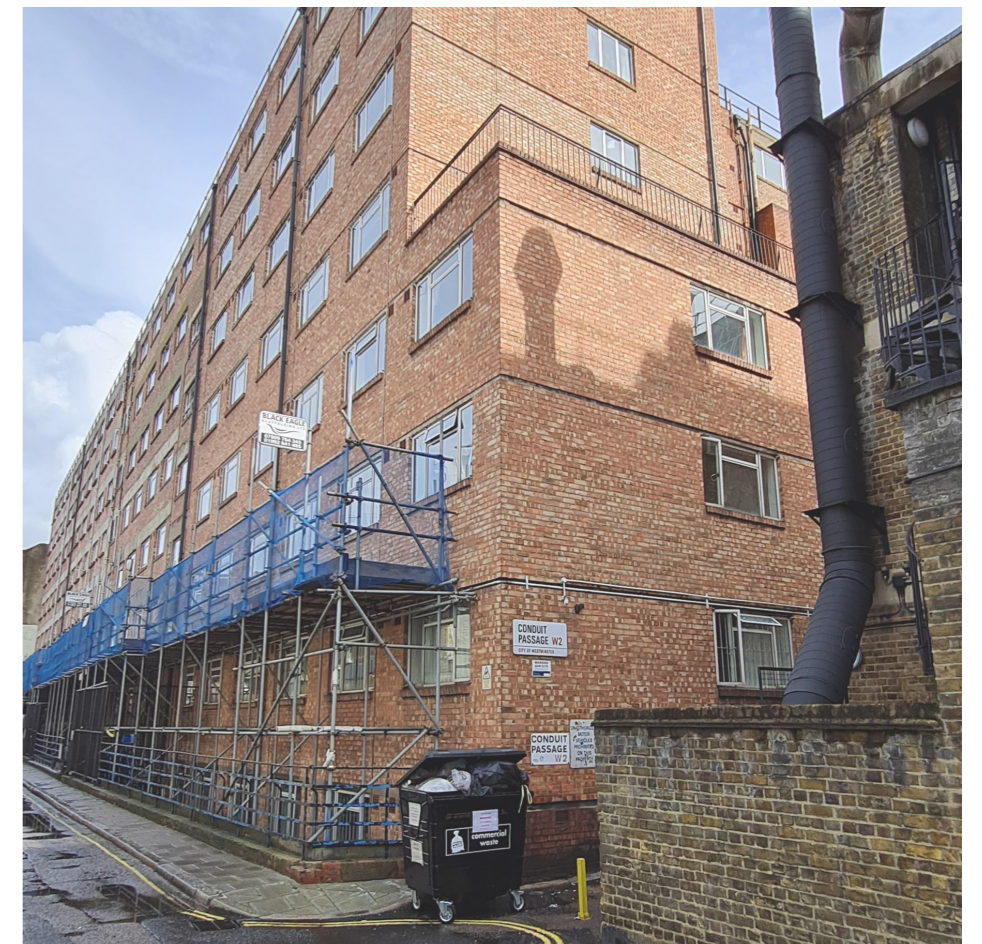
4. View from Conduit Place
