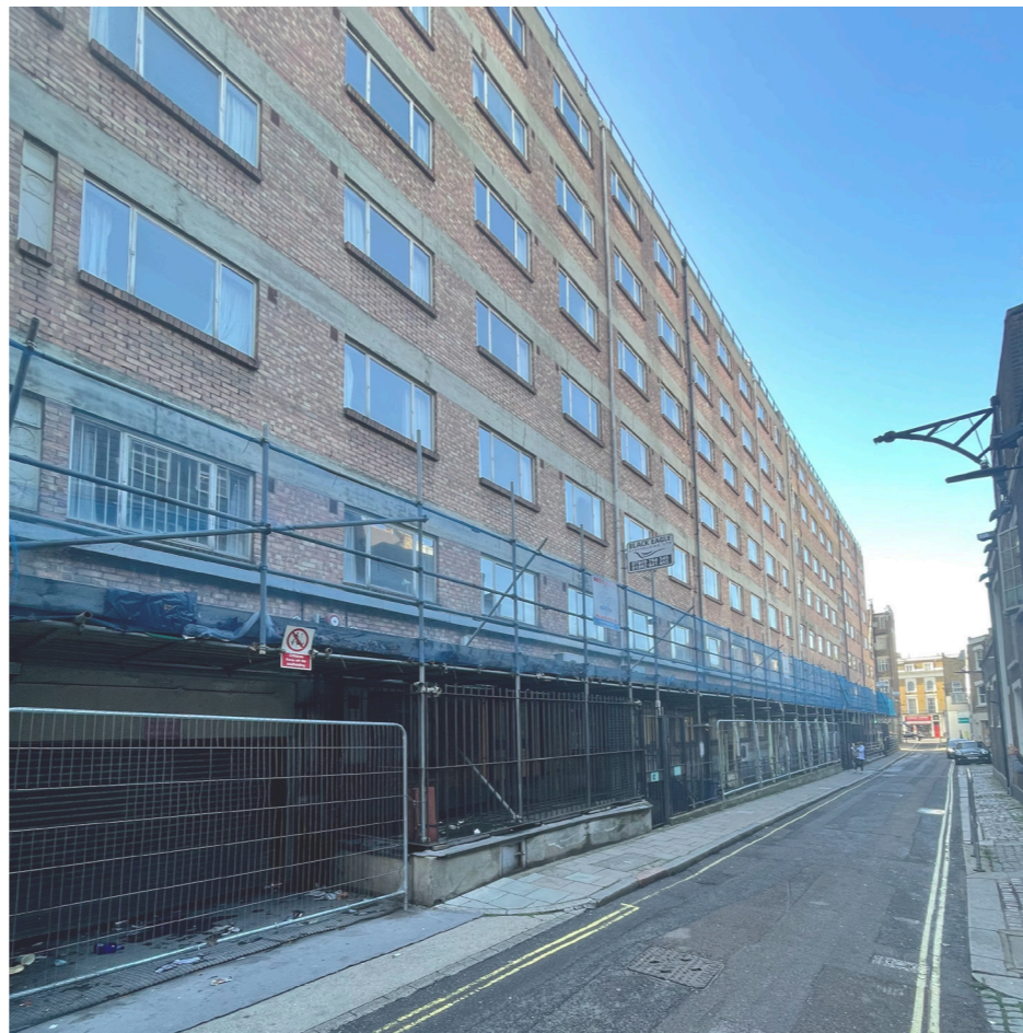
3. View from Conduit Place
