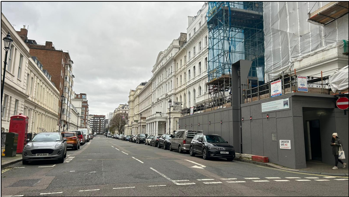
Photograph 1 – View from Lancaster Gate towards the entrance to the site.
