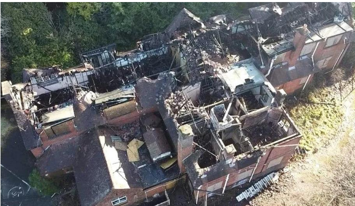
Photograph 2 – Aerial view showing the extent of the fire damage to Broughton House (photo supplied by BCP Council)
