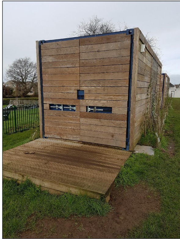
Typical container cladding
