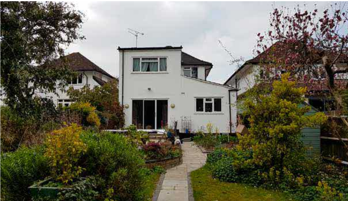
Photo 3 - Rear of the house before the current ongoing construction work
