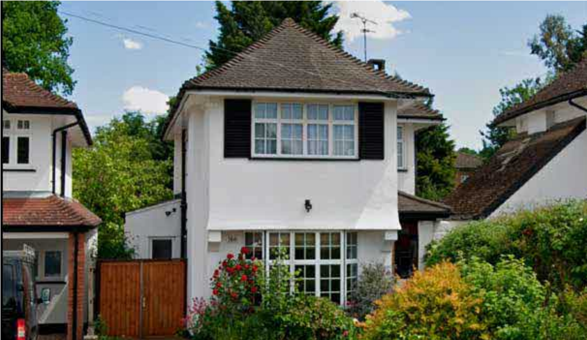
Photo 2 - Front of the house before the current ongoing construction work
