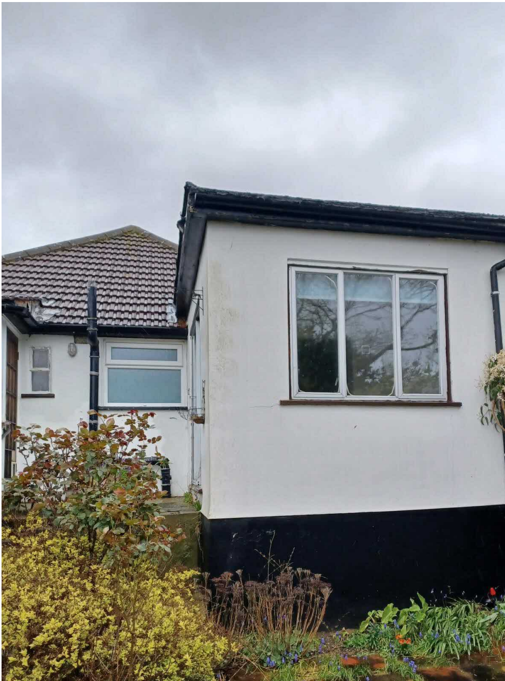
Rear elevations showing the existing single storey extension
