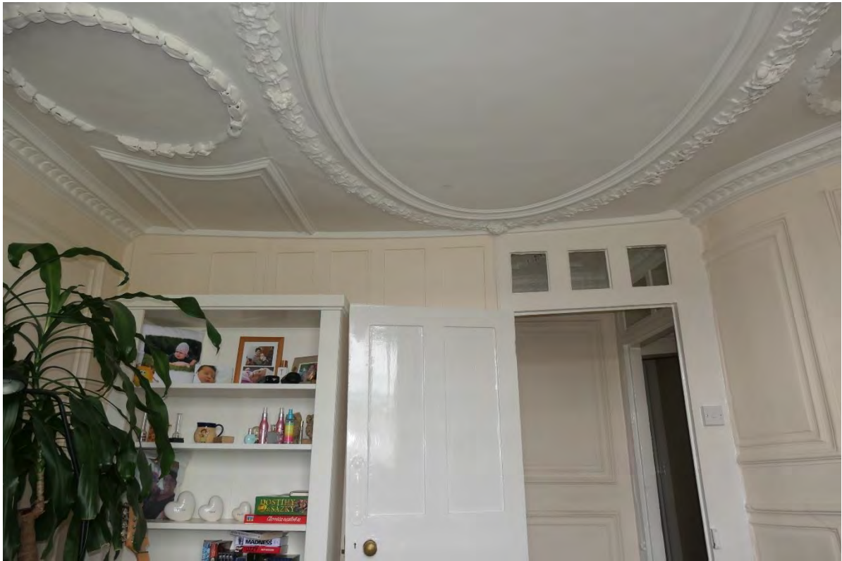
Photo 14: The central first floor front room, looking south towards the inserted wall that cuts across the ceiling and which now forms corridor along the south.
