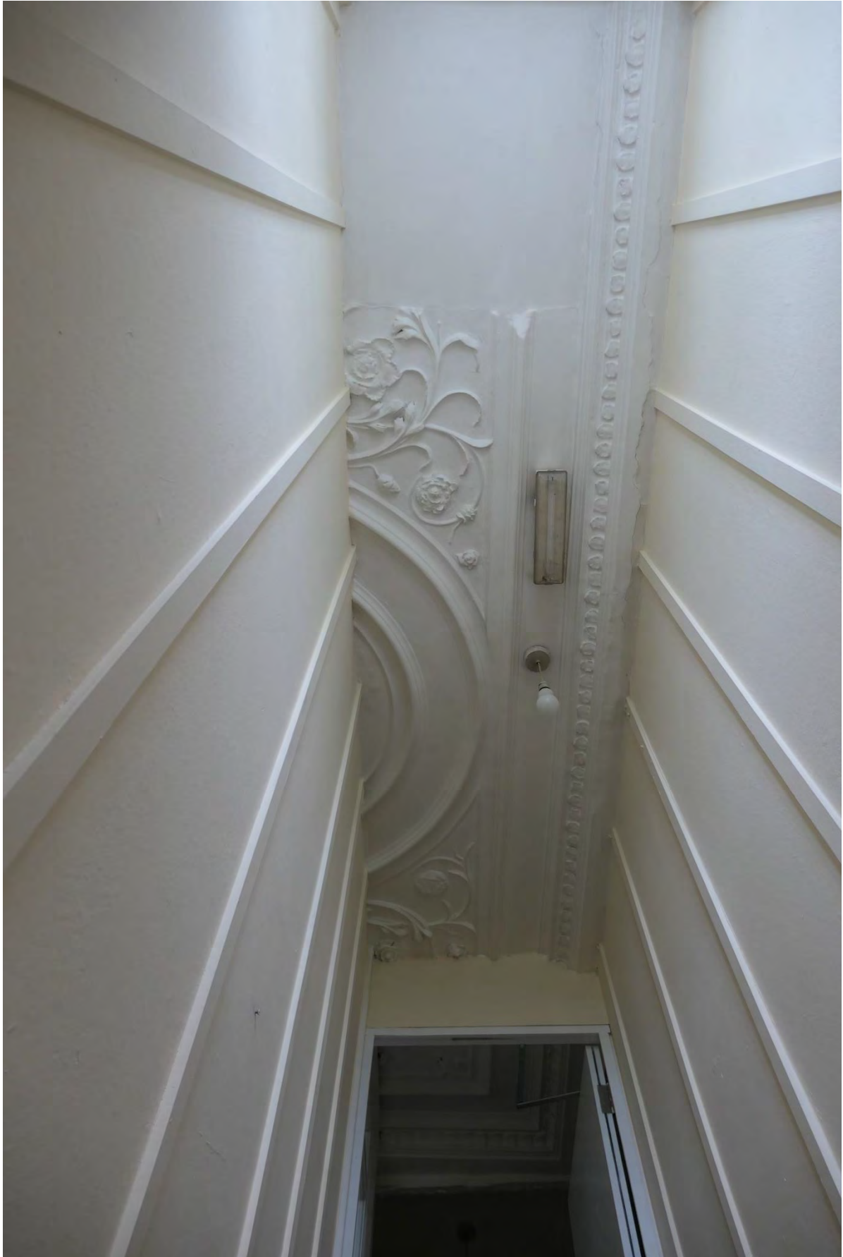
Photo 10: The ground floor, seen from the front room, looking towards the rear.
