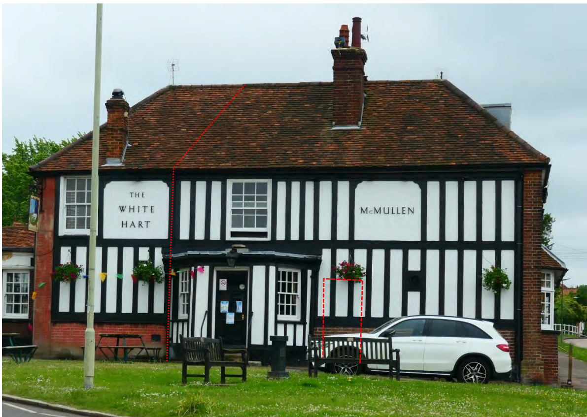
Photo 1: A frontal view of The White Hart, with the red dotted line showing the likely line of the eastern extension, with an original arrangement of a central stack heating two rooms and lobby entrance (approximation shown in dotted red line).
