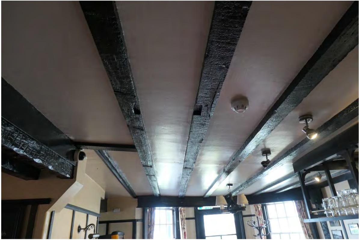
Photo 6: The re-used joists.
