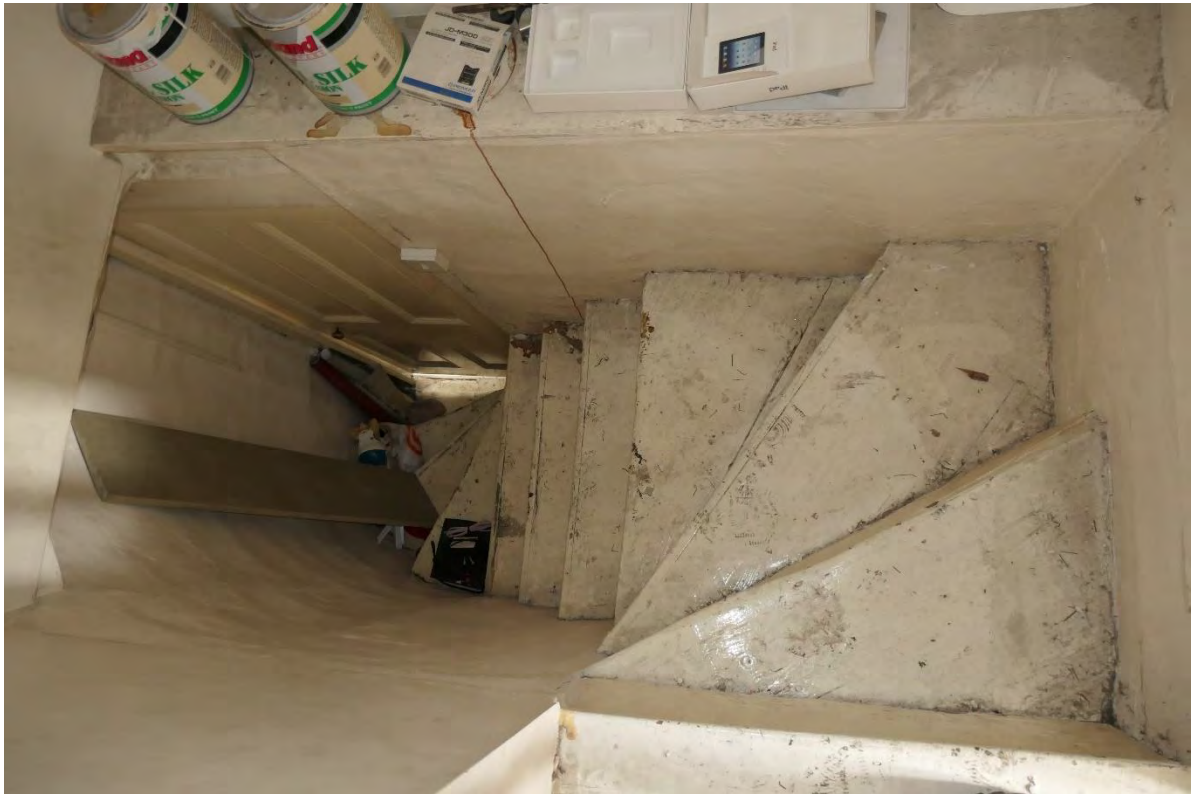
Photo 23: The curved little staircase to the roofspace looks to be original.
