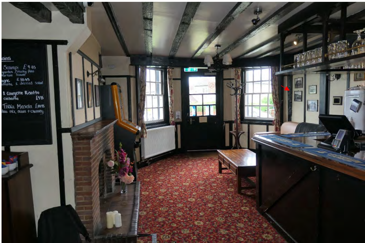
Photo 5: The central front room of The White Hart. The C20 fireplace can be seen on the left, and a timber post on the right is shown with a red arrow. The narrow, widely spaced and long span re-used joists appear to be primarily decorative, rather than structural.
