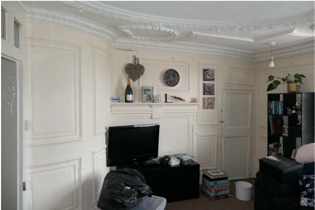
Photo 17: The west wall with chimneypiece in the central first floor front room.
