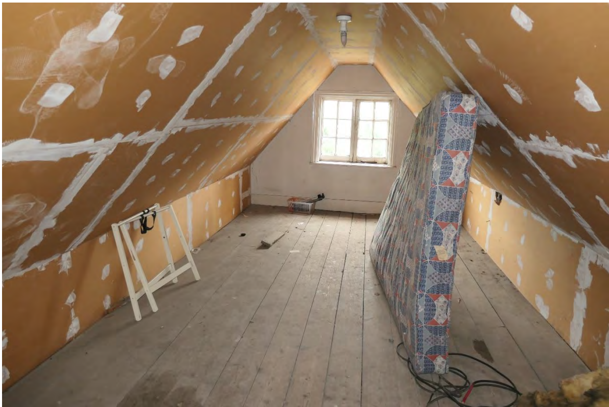
Photo 24: The roofspace has been dry-lined and the structure is not exposed.
