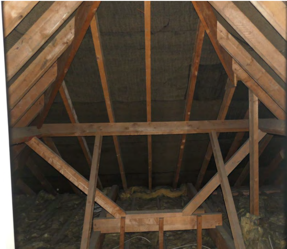
Photo 24: Where the structure is exposed, it is of no great age.
