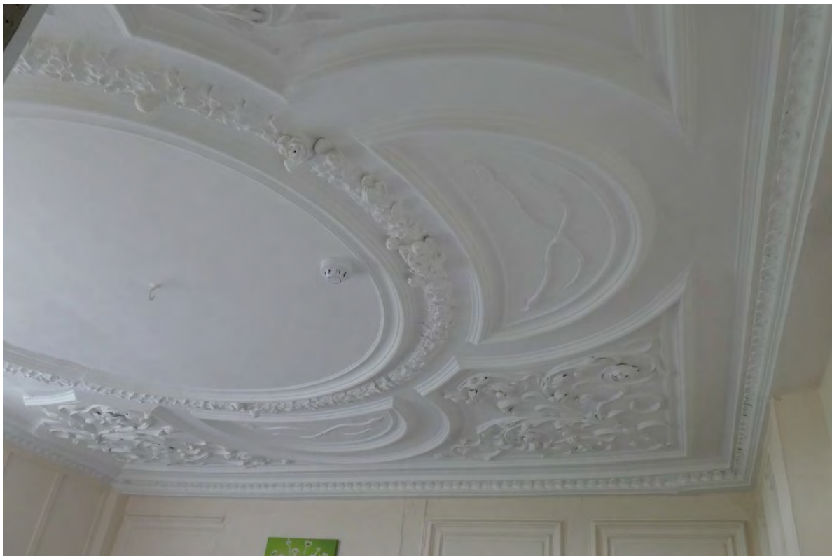
Photo 11: The ceiling in the NW first floor room.
