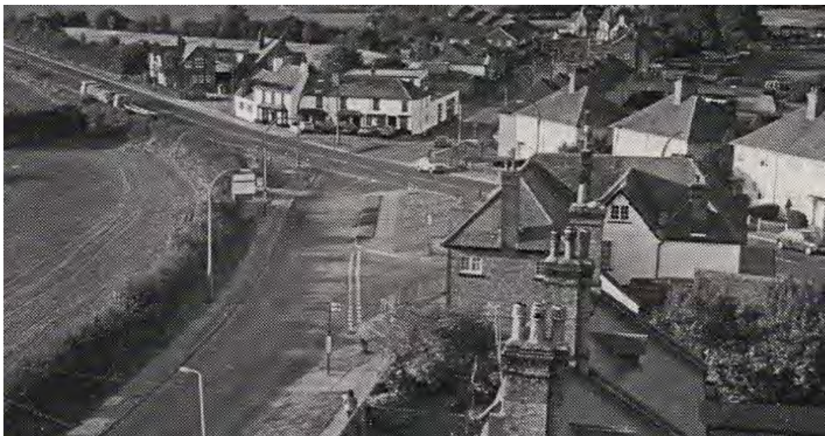
Fig 14: An extract of an elevated c. 1970s photo of The White Hart from the south.
