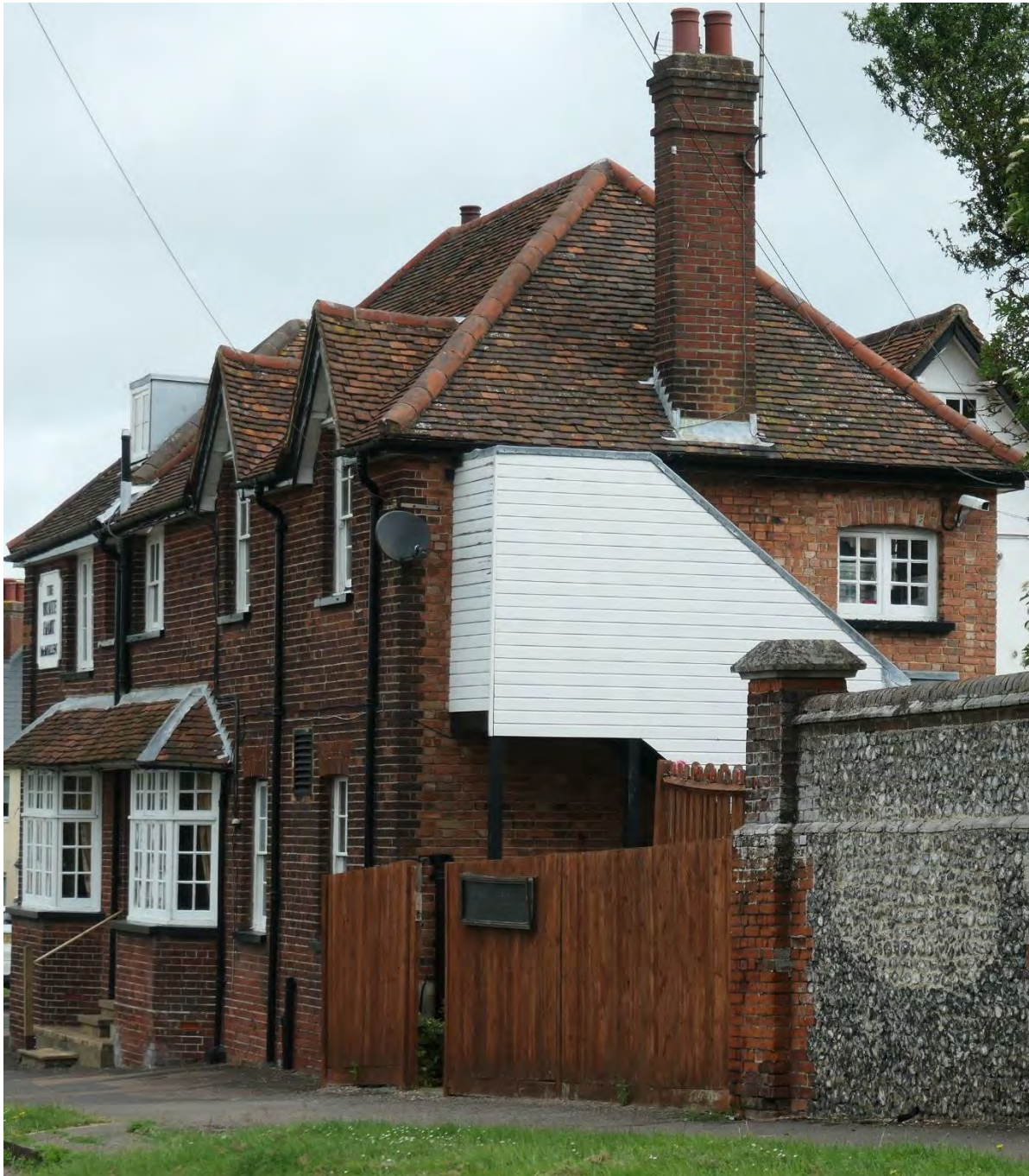
Photo 29: The existing poor quality staircase and 'Fletton' brick wall.
