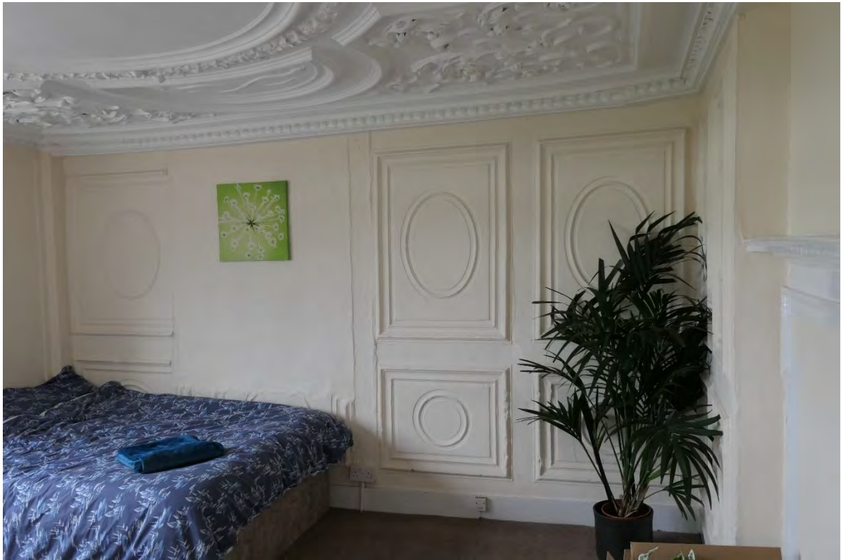
Photo 12: The plaster wall panels in the NW first floor room.
