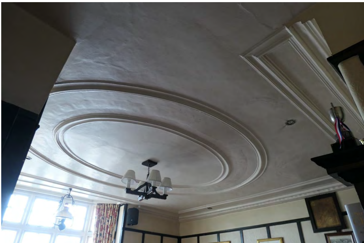
Photo 9: The plaster ceiling to the NE ground floor room.
