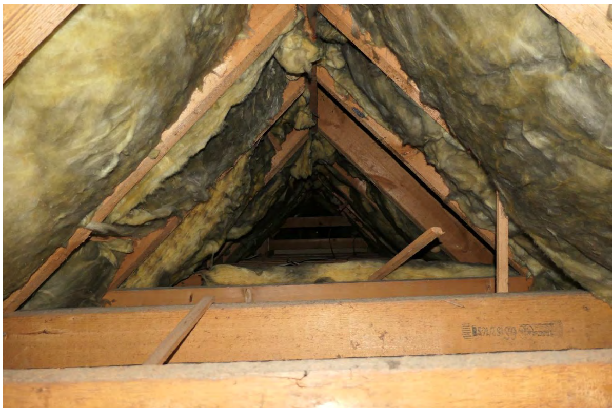
Photo 25: Where the structure is exposed, it is of no great age (the timbers seen here are modern).
