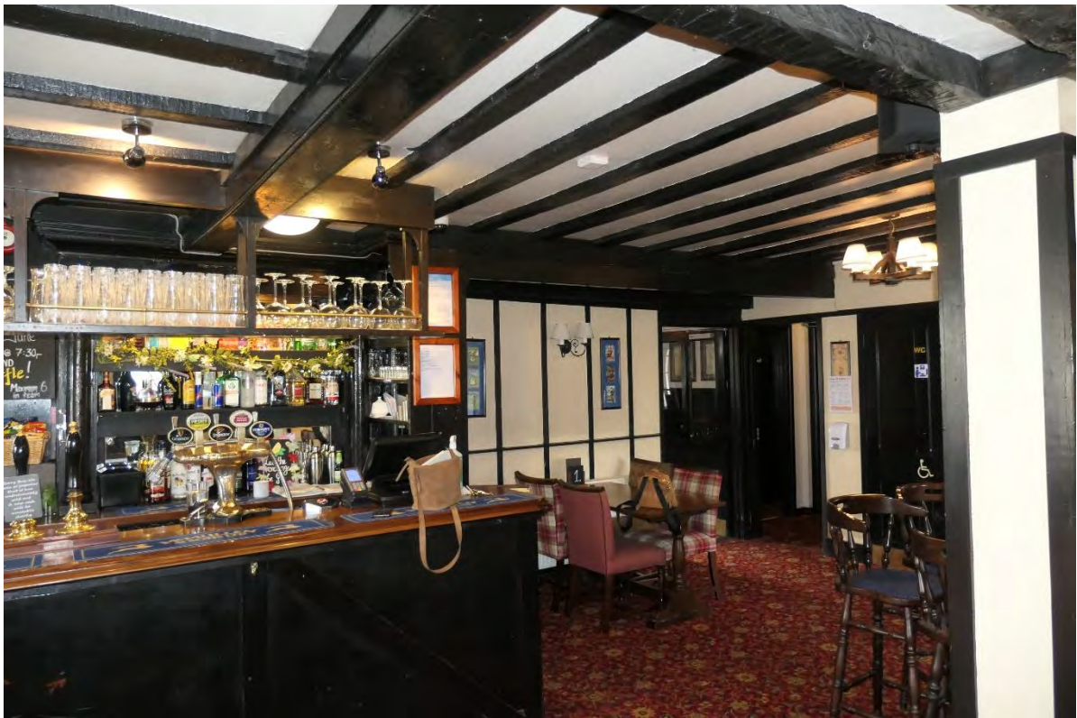
Photo 7: The joists at the central rear room of The White Hart.
