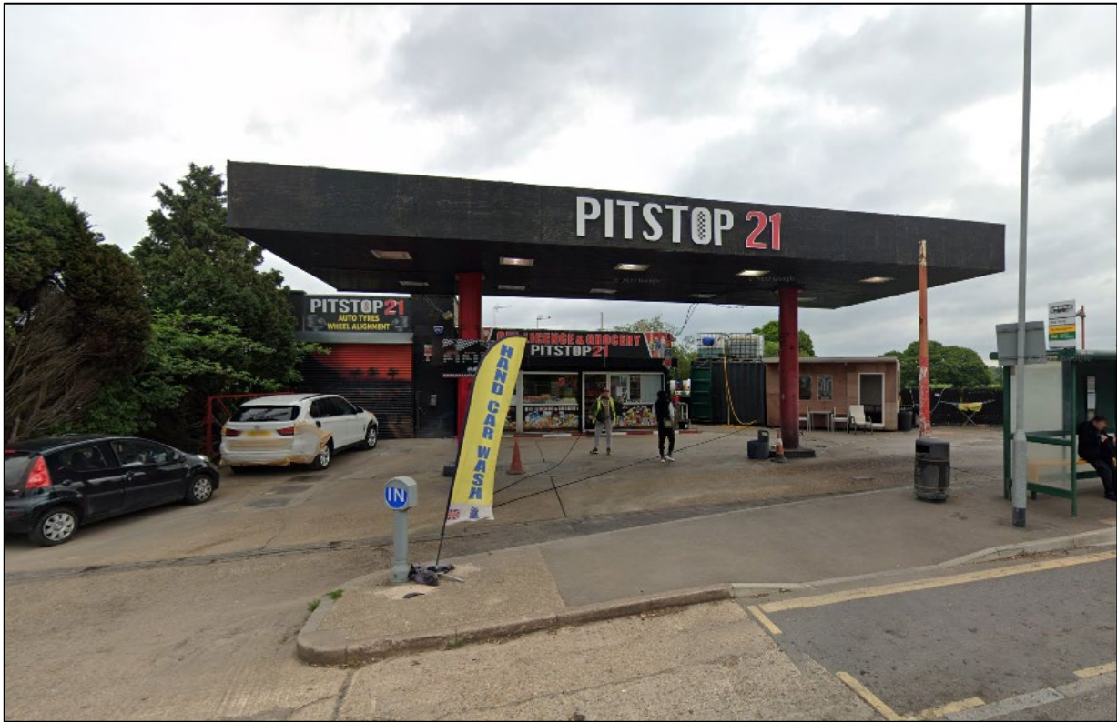
Figure 7: Convenience Shop and Car Wash (Google Streetview)
