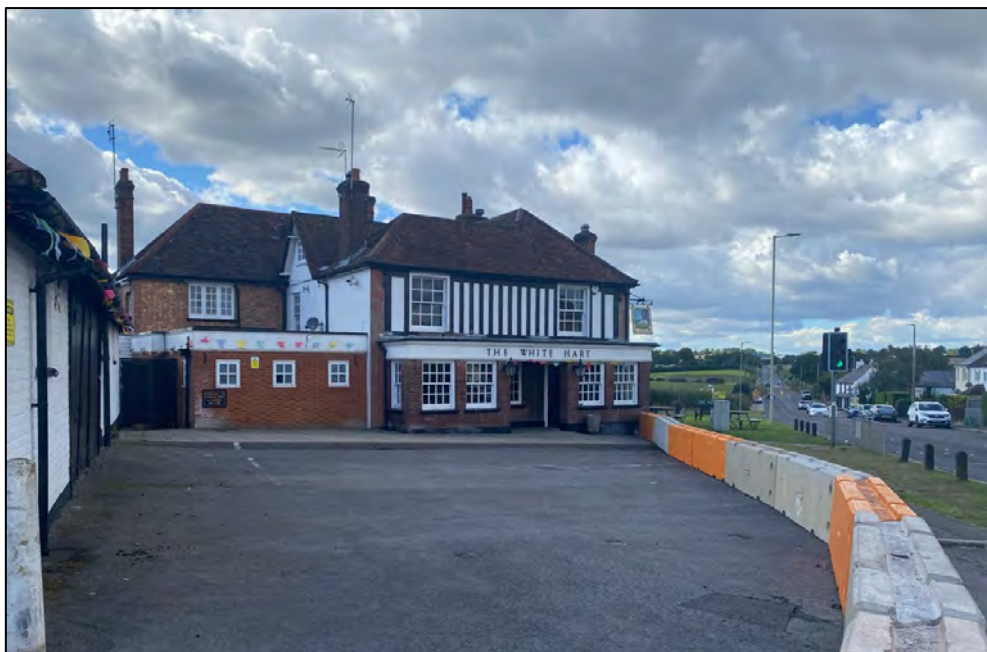
Figure 2: Streetview of the application site from the B556, looking north-west from the access.
