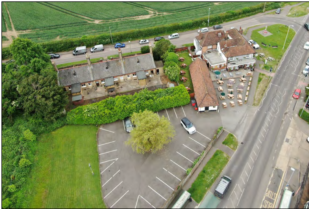
Figure 4: Aerial view of the application site, looking north-west over the site.
