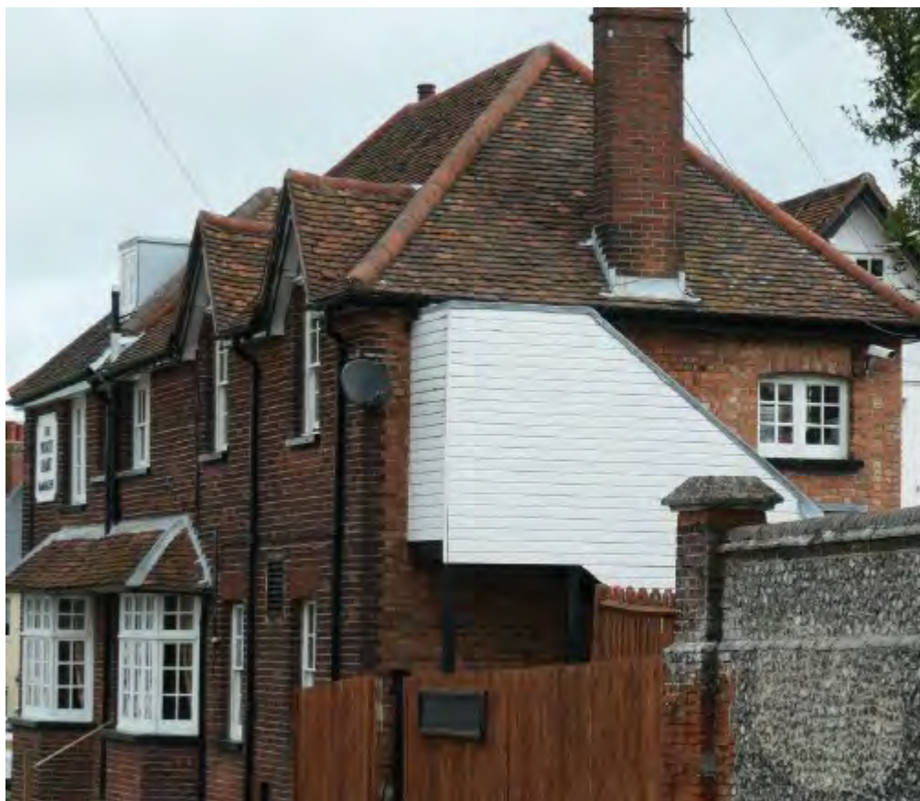
Figure 11: Modern extensions to the building.
