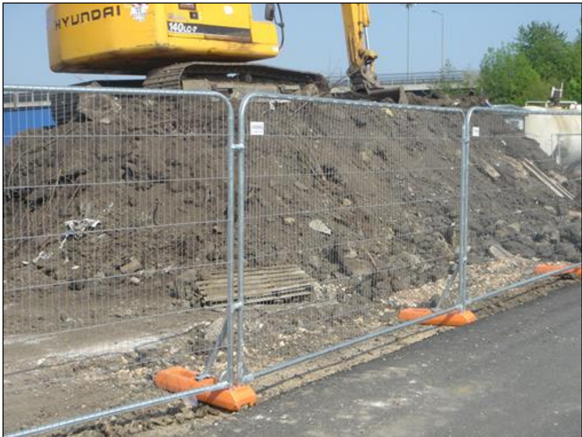
Photograph F – Example of Heras Tree Protective Fencing
