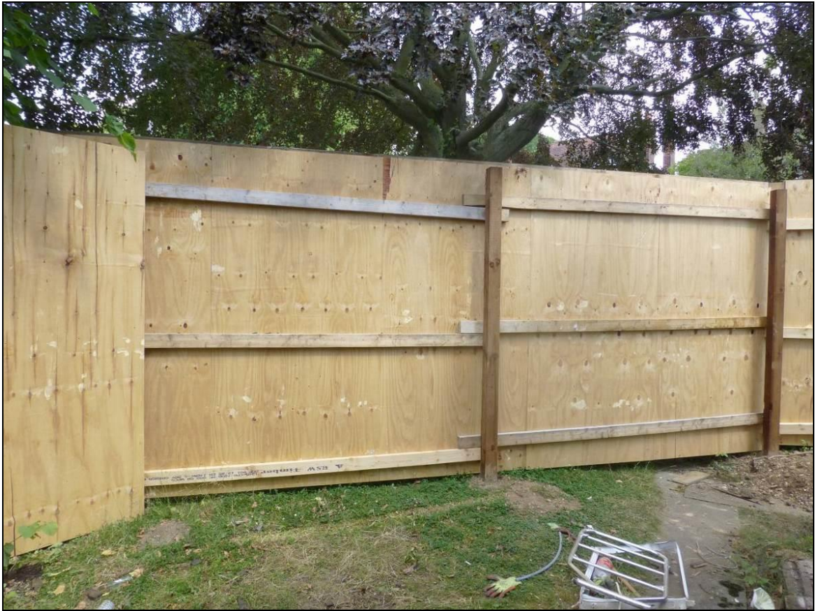
Photograph E – Example of Timber Hoarding Tree Protective Fencing.
