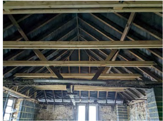
Photograph 4. Interior of B2.
