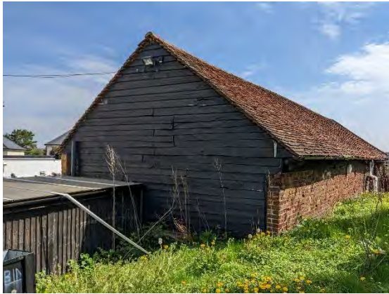
Photograph 3. Western aspect of B2a (storage building).
