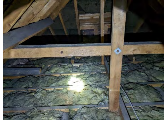
Photograph 2. Loft void in B1.
