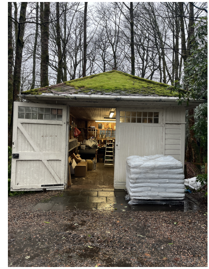
(Photo of existing)
