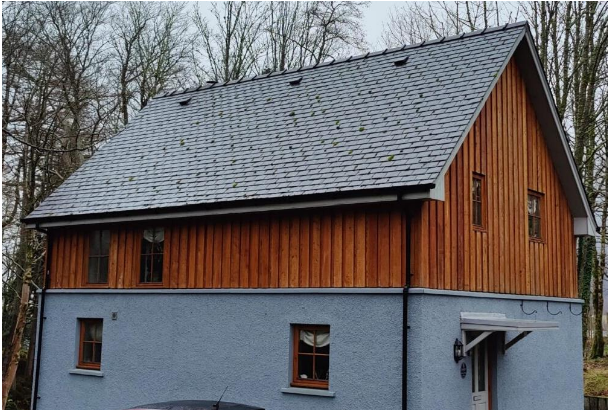
15) View of Bishop's Bay Cottage Roof in natural stone slate, as is being proposed for the shed.
