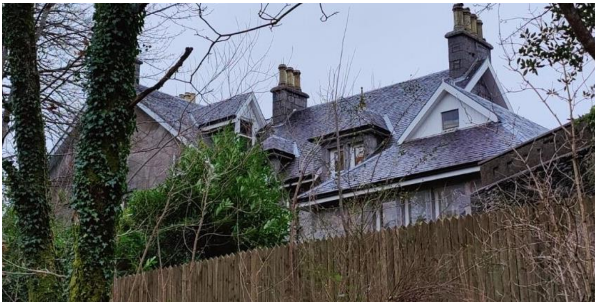
16) View of the Alltshellach Hotel building nearest to Bishop's Bay cottage, showing a natural stone slate roof, also used on all of the other hotel buildings.
