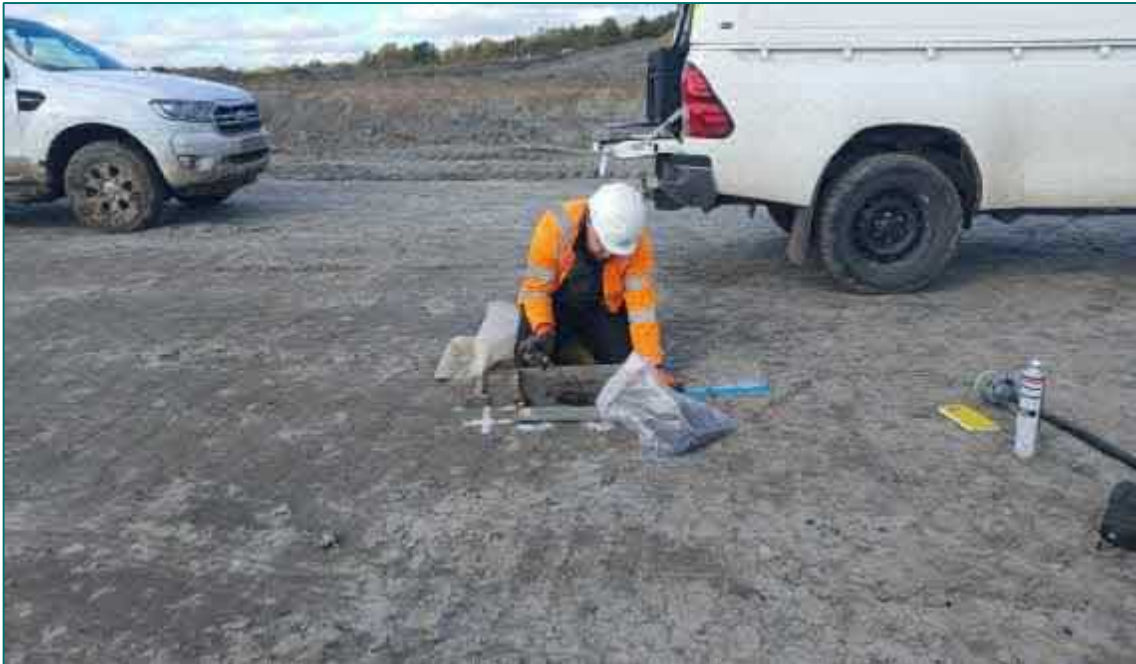
Photograph 9 –Earthworks: Validation Testing on Compacted Layers (Sand Replacement Test)
