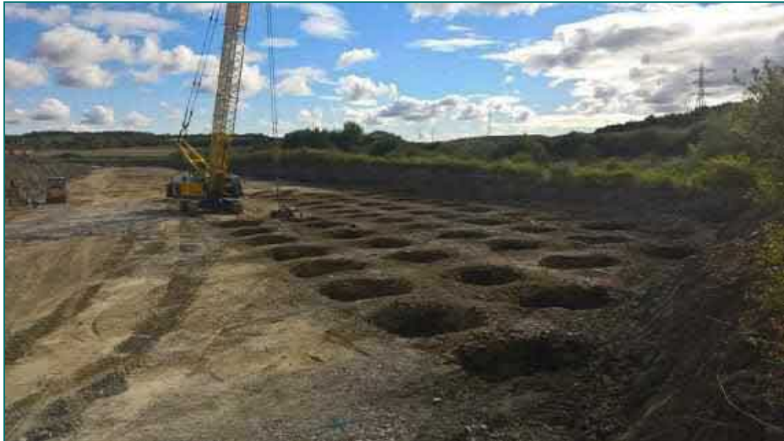
Photograph 5 –Dynamic Compaction
