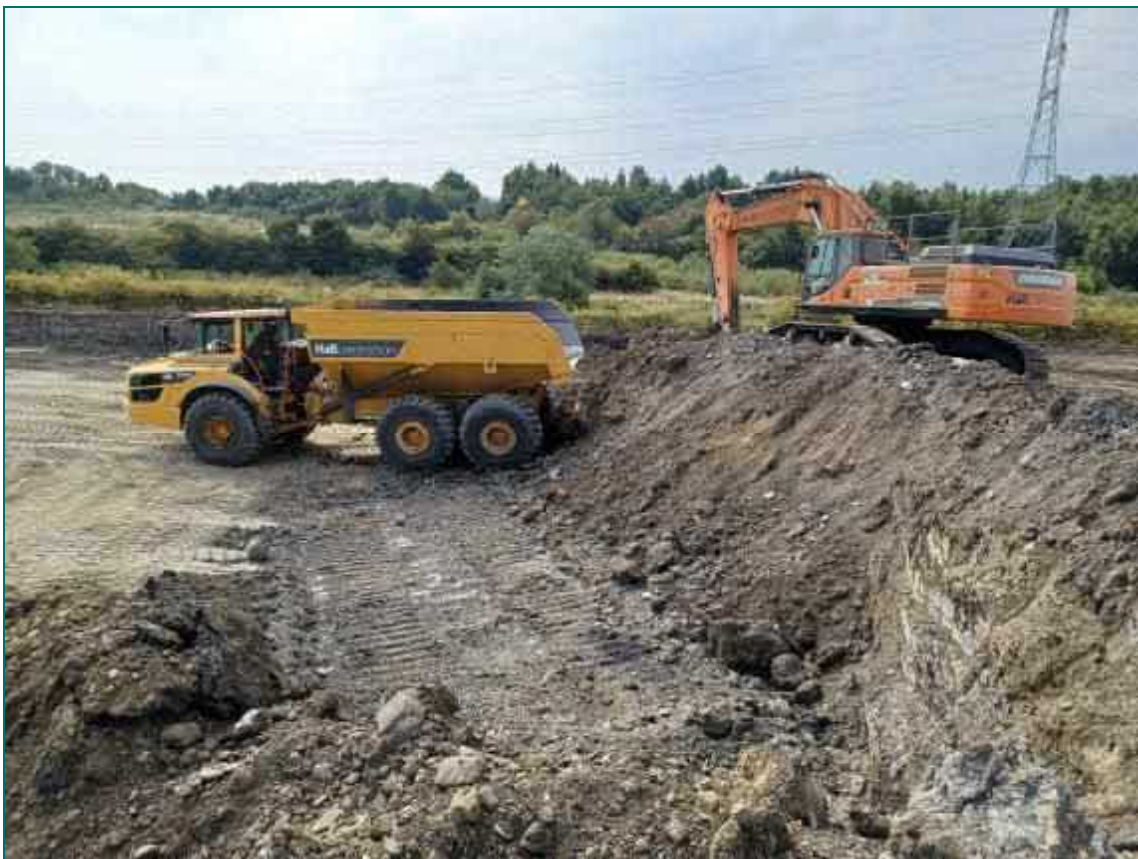
Photograph 2 –Excavating the Cuts to Dynamic Compaction Level
