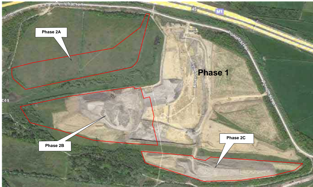
Figure 1 Site plan of the Skelton Grange development with Phase 2A, 2B and 2C highlighted by red line boundaries.
