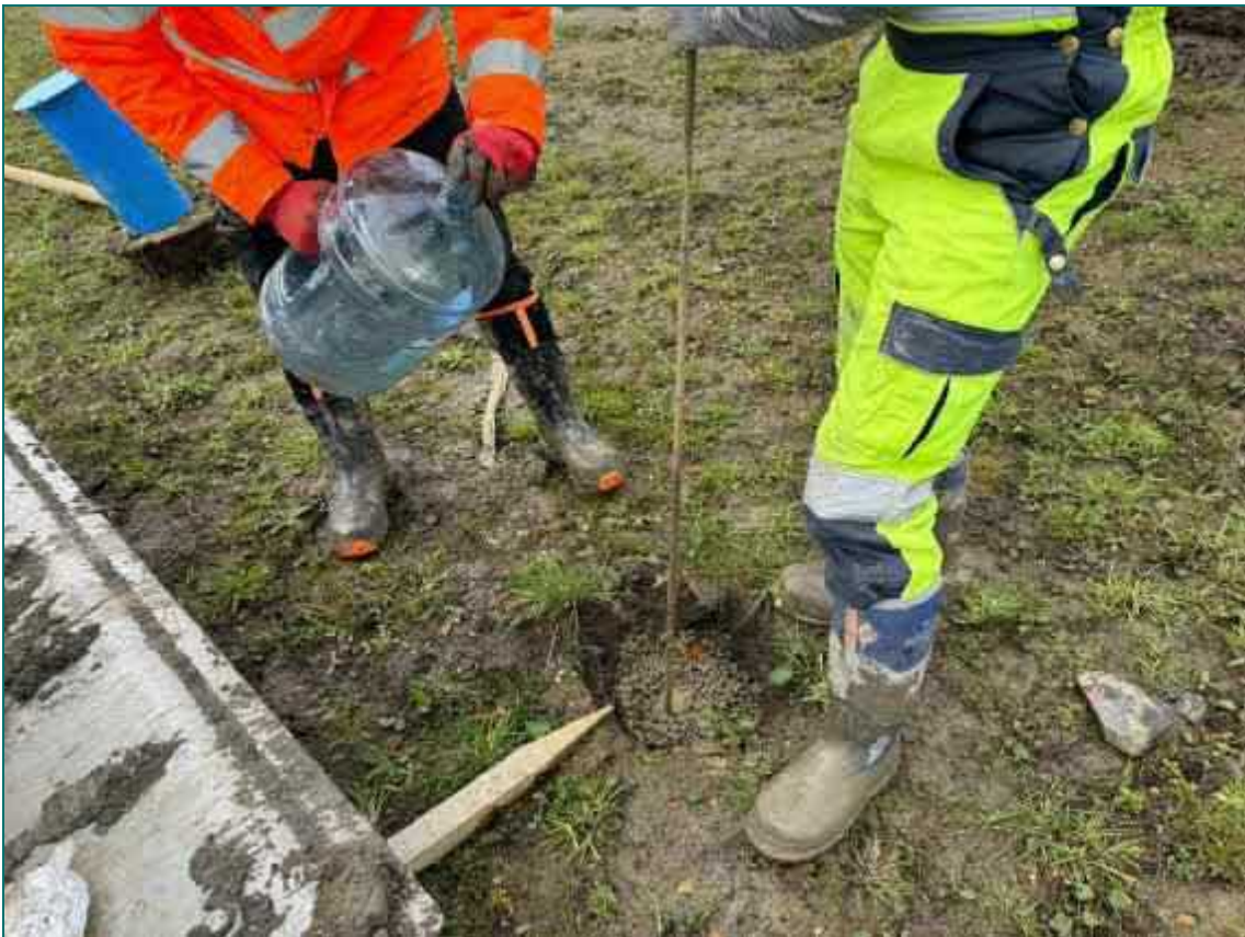
Photograph 15 –Decommissioning of Shallow Ground Gas Wells
