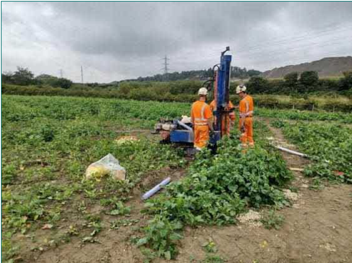
Photograph 13 –Installation of Monitoring Wells for Post Earthworks Continuous Gas Monitoring
