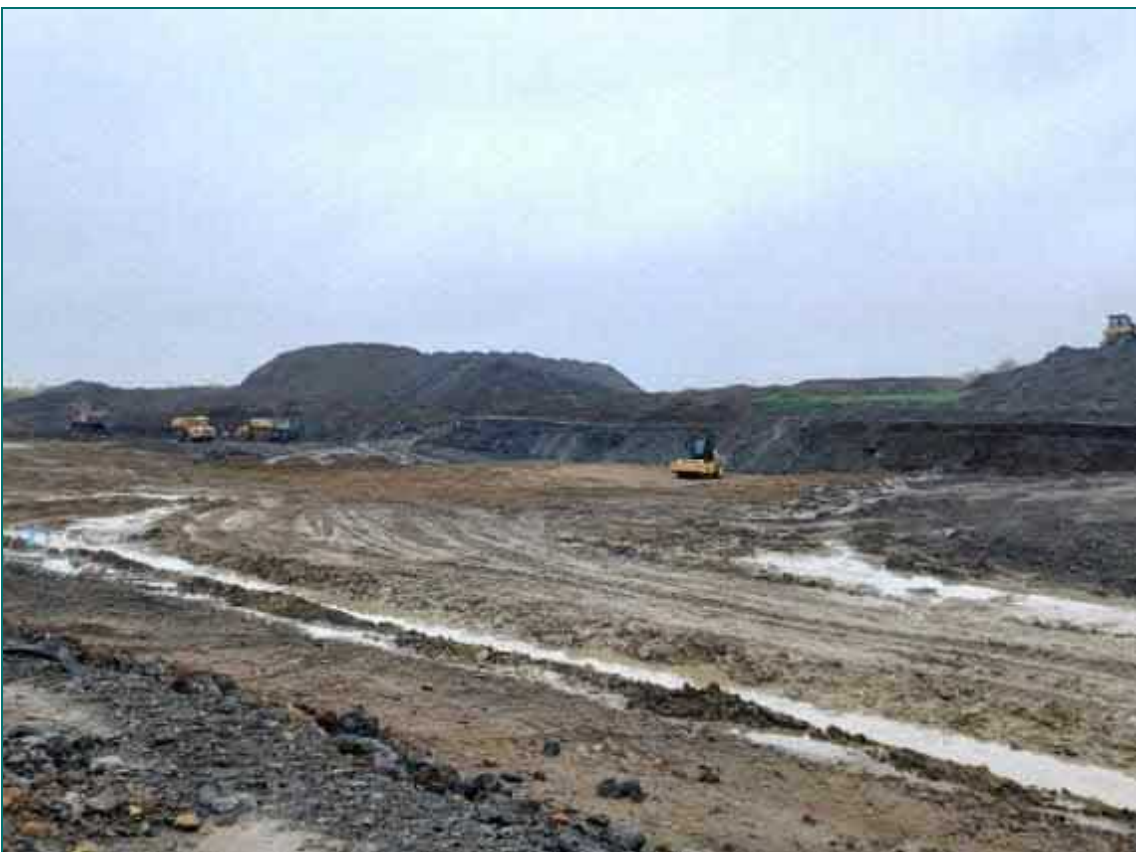
Photograph 4 –Temporary Drainage Channels to Allow Works to Continue During Wet Weather
