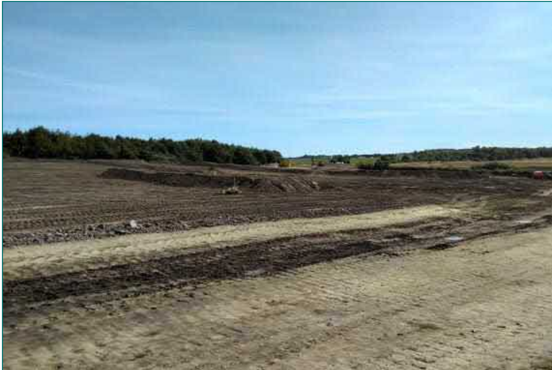
Photograph 1 –Topsoil Strip
