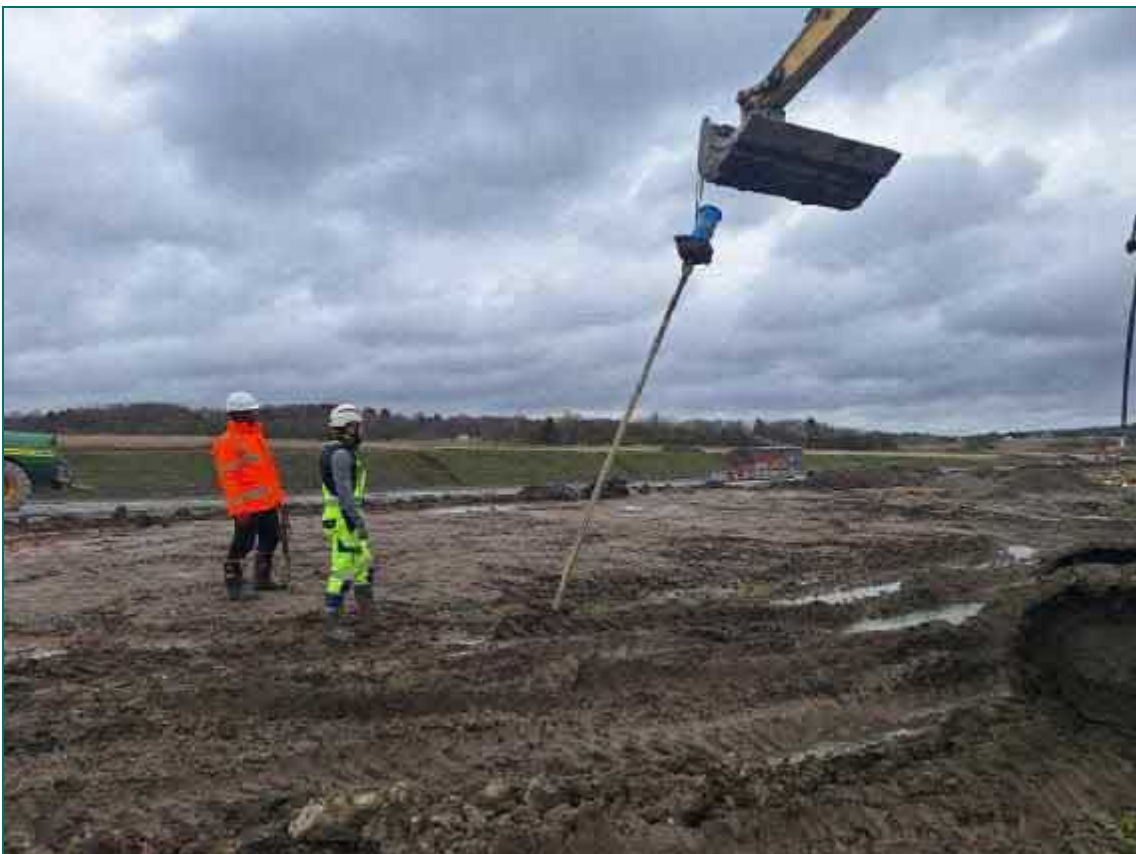
Photograph 14 –Decommissioning of Shallow Gas Monitoring Wells
