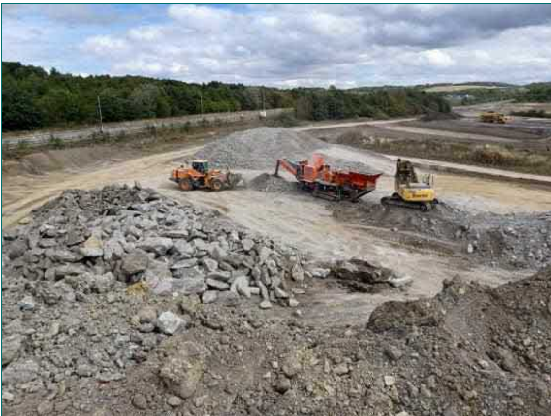
Photograph 10 –Crushing of Sandstone Boulders
