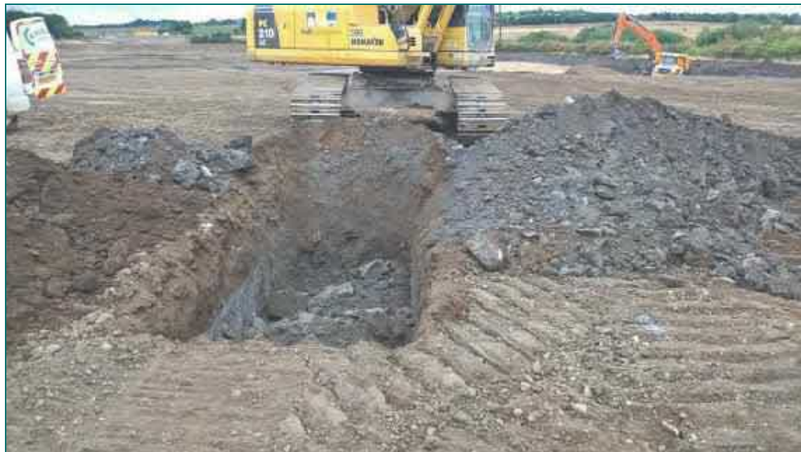
Photograph 6 –Trial Pits to Obtain Representative Soil Samples for Laboratory Classification
