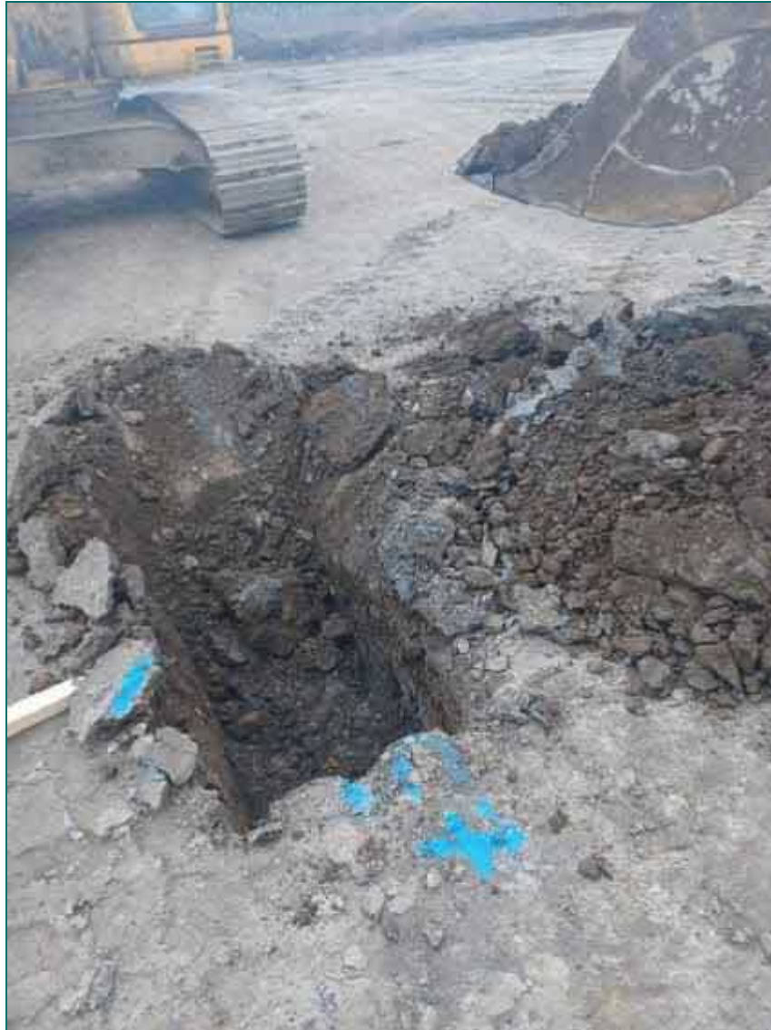
Photograph 12 – Trial Pits for Chemical Validation on 50m Grid.
