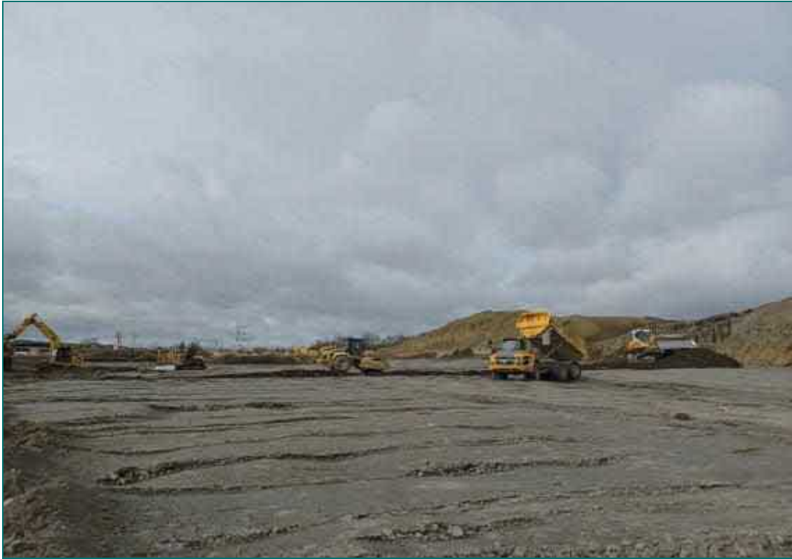
Photograph 7 –Earthworks: Engineering of Class 2C Materials
