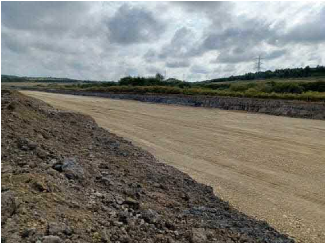
Photograph 3 -Dynamic Compaction Platform on Cut 2B3
