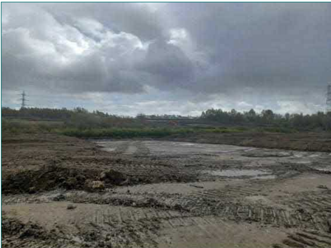
Photograph 11 –Replacement of Topsoil, Excluding area for Pedestrian Bridge Construction
