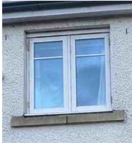
TYPICAL EXISTING WINDOW (WINDOW 3)
