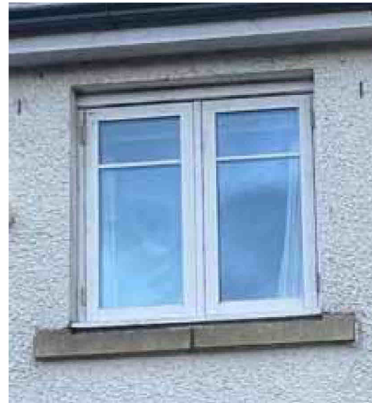
TYPICAL EXISTING WINDOW (WINDOW 3)
