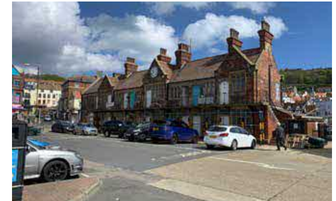
Building 1 - View from the Car Park
