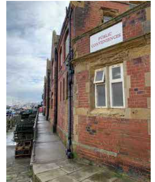
Building 1 South East Elevation
