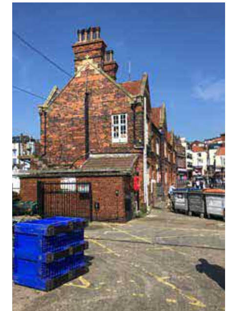
Building 1 South East Elevation
