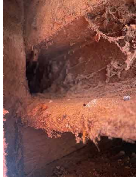
Figure Men's toilet location 8
