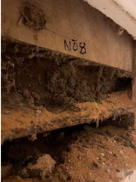
Figure Men's toilet location 8
