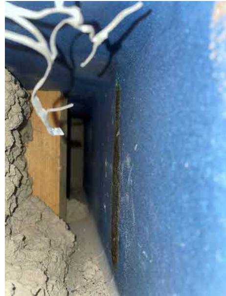
Figure Women's toilet location 5
