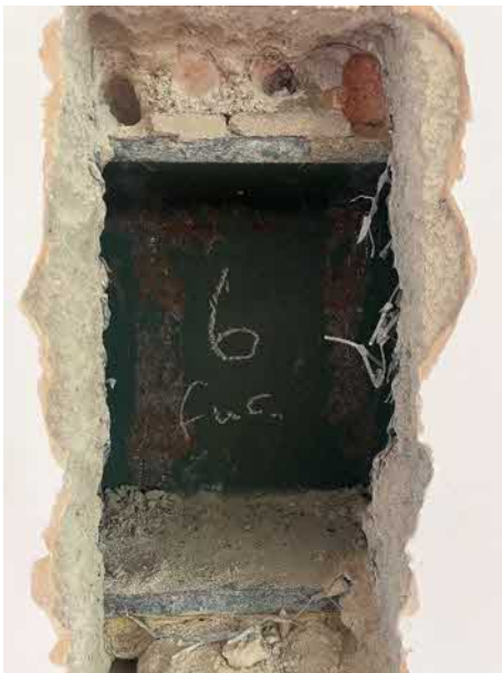
Figure Women's toilet location 6
