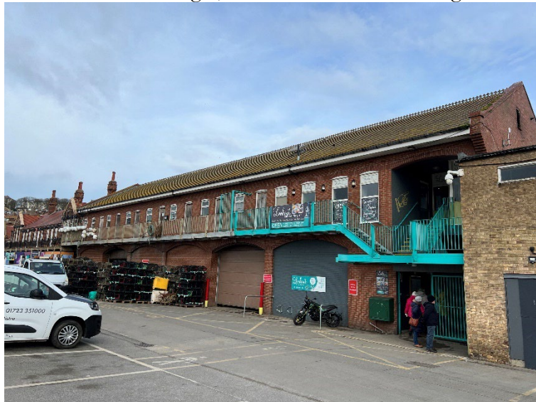
Plate 8 – Building 3, west elevation and south gable.
