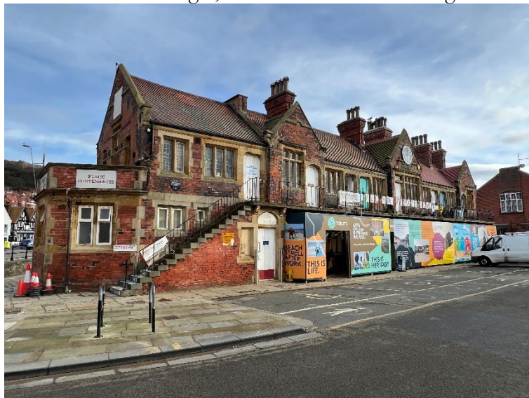
Plate 3 – Building 1, west elevation and north gable.
