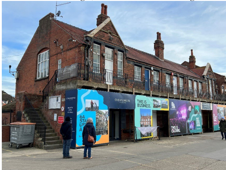
Plate 5 – Building 2, west elevation and north gable.
