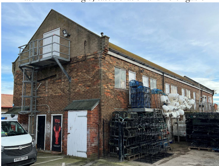
Plate 12 – Building 5, east elevation and north gable.
