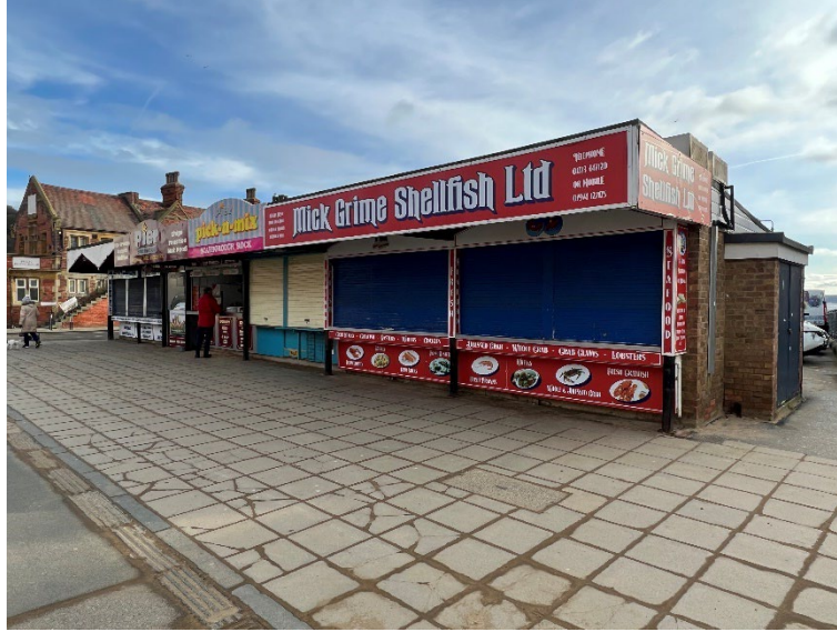
Plate 1 – Kiosks (Building 6), north and west elevation.
