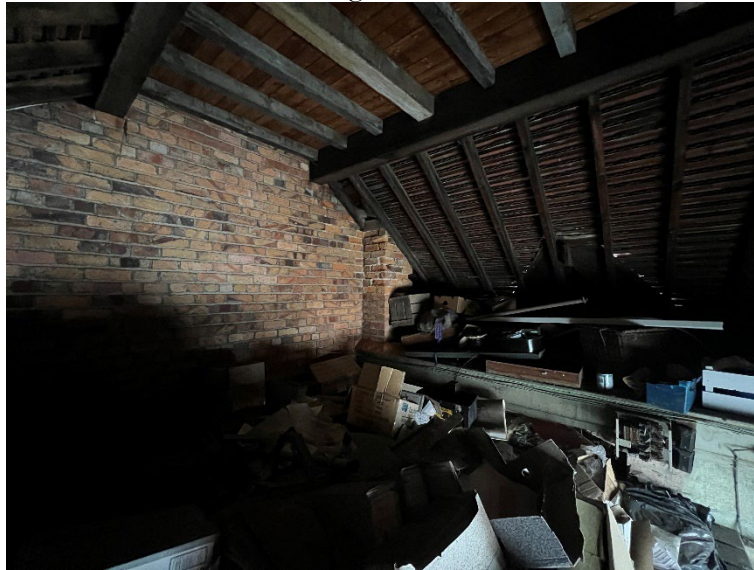
Plate 7 – Building 2, internal roof void.
