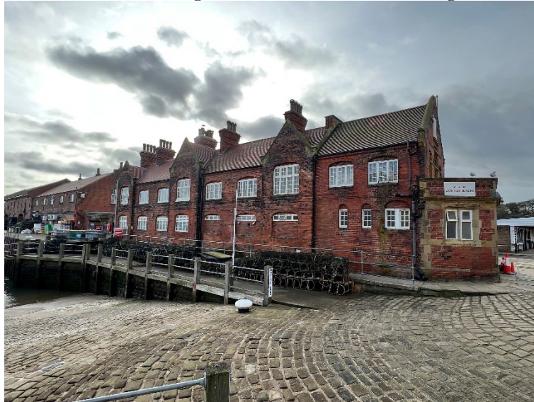
Plate 2 – Building 1, east elevation and north gable.
