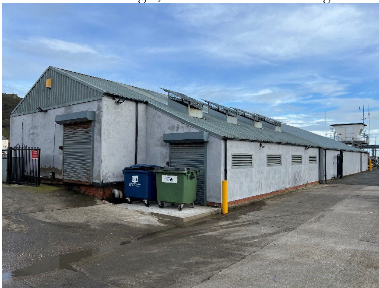
Plate 10 – Building 8, west elevation and north gable.
