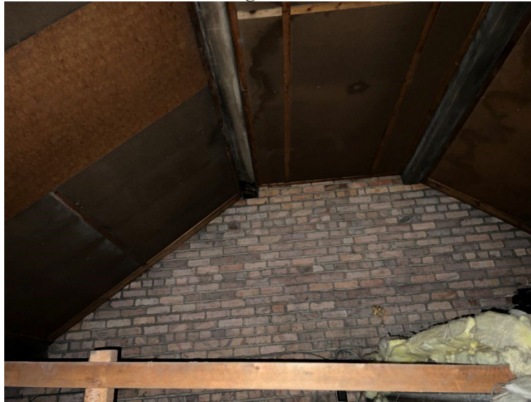
Plate 4 – Building 1, internal roof void.
