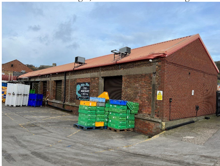
Plate 9 – Building 4, west elevation and south gable.
