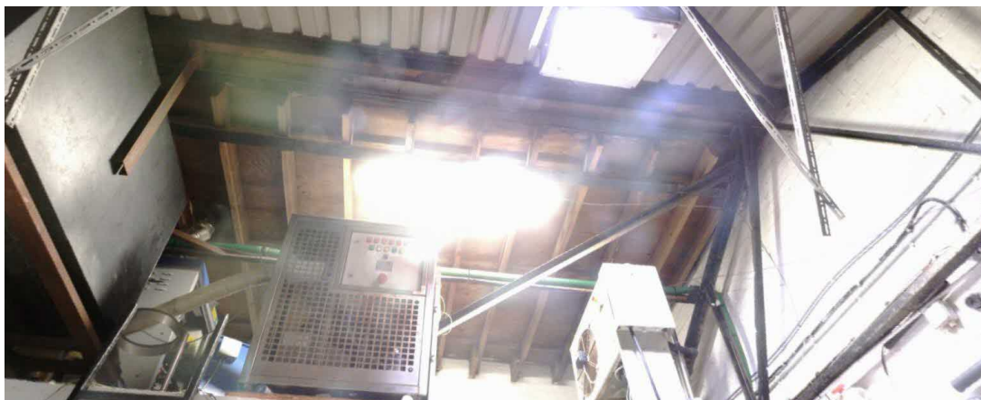
Figure 3 Building 4b Timber Roof Deck Spanning onto Purlins of Building 4a
