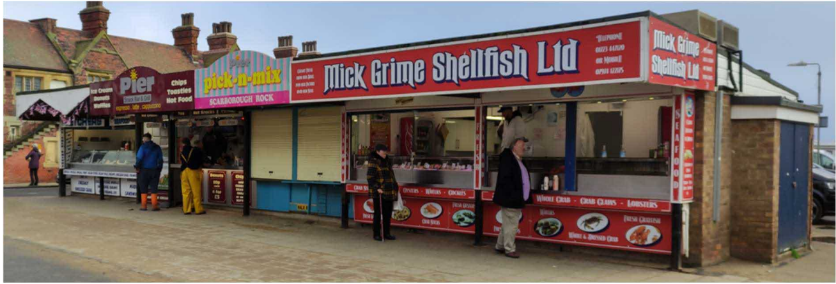
Photo 16 - North-west elevation of Kiosks
