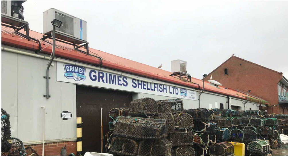
Photo 3 - North-east elevation of Building 4a adjacent to Building 3
