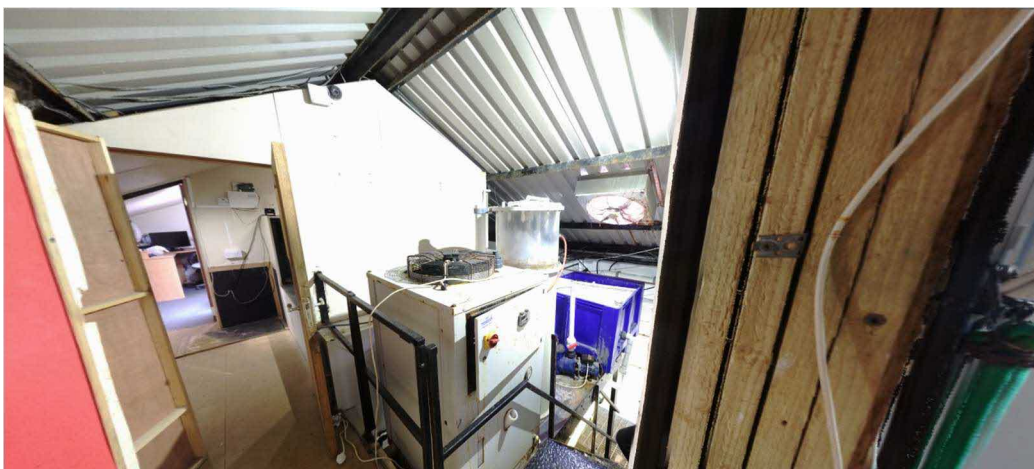
Photo 5 - Steel staircase to loft of Building 4a
