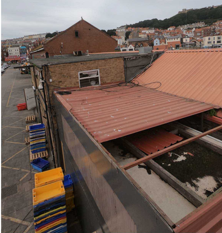
Photo 12 - Aerial perspective of Building 4c Roof
