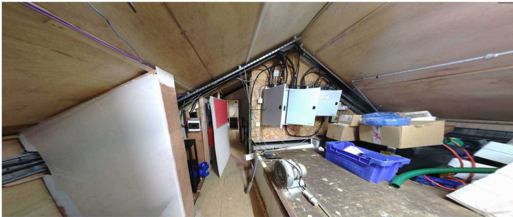
Photo 4 - Converted loft space of Building 4a
