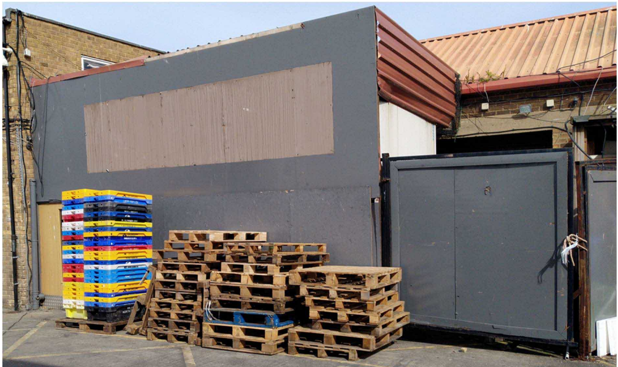
Photo 11 - South-west elevation of Building 4c
