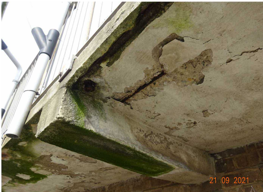
Photo 15 - Reinforced concrete basement present along south-east elevation of Building 7
