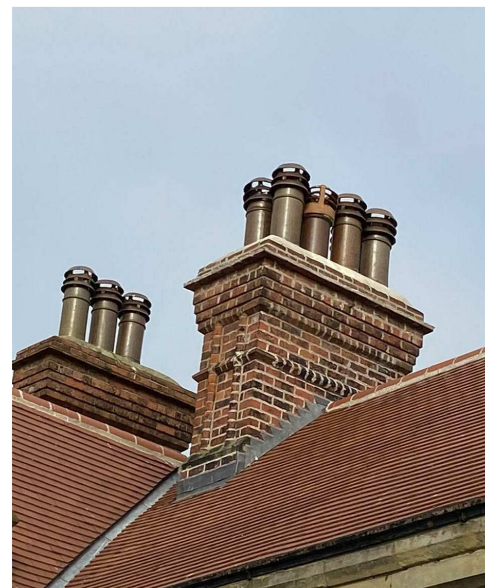
Example condition of Chimney
