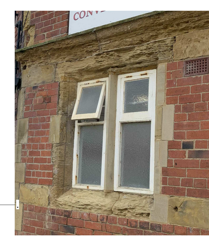
Condition of existing stone window surrounds and feature banding
