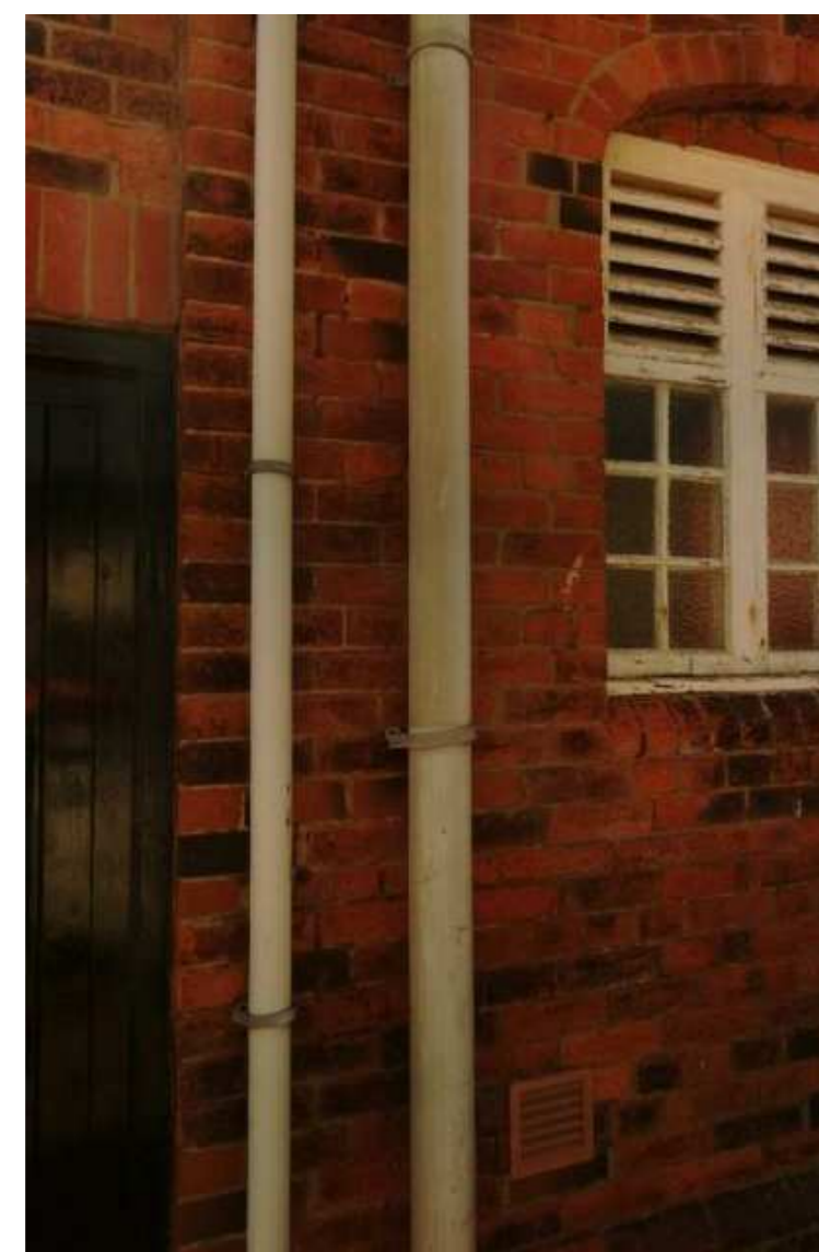
Example of uPVC Rainwater Goods to be replaced/removed with Cast Iron
