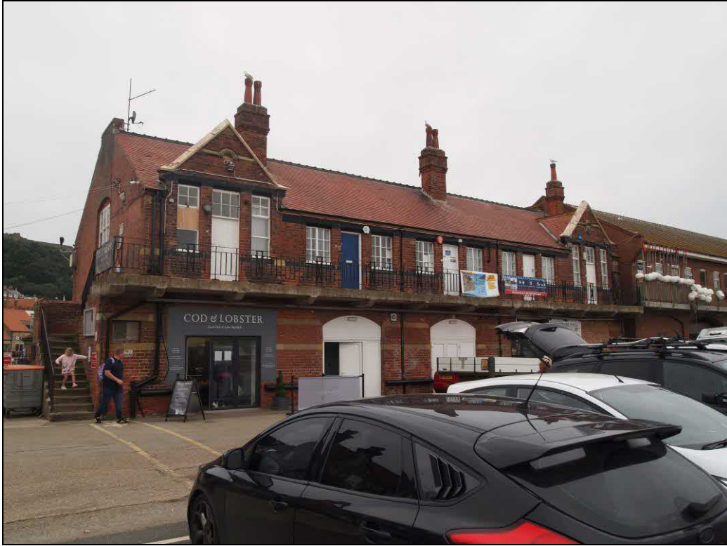
Figure 9: Building 2 front elevation.
