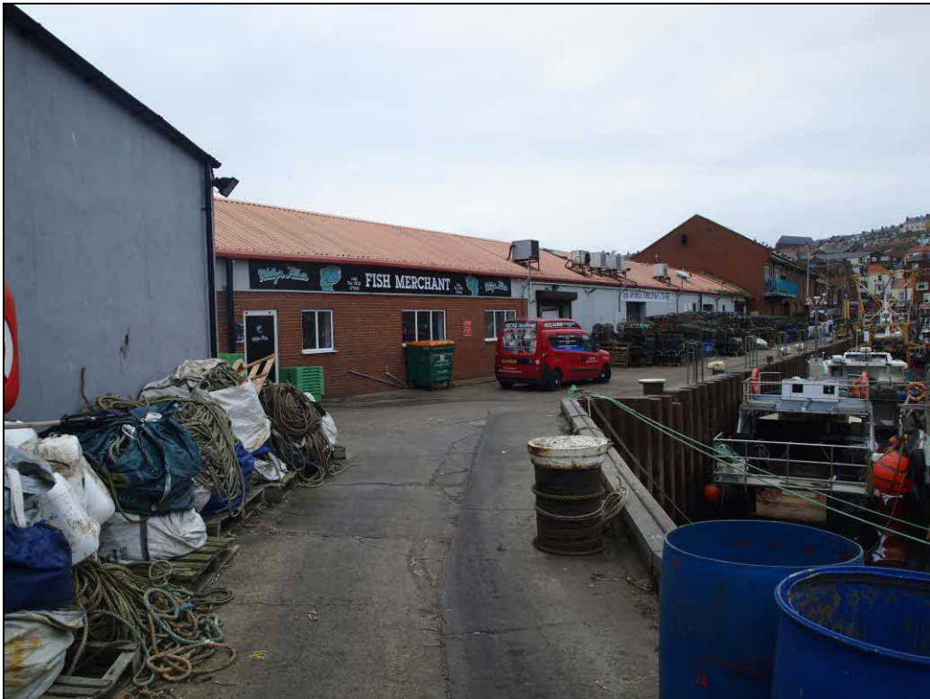
Figure 12: Building 4 rear elevation.
