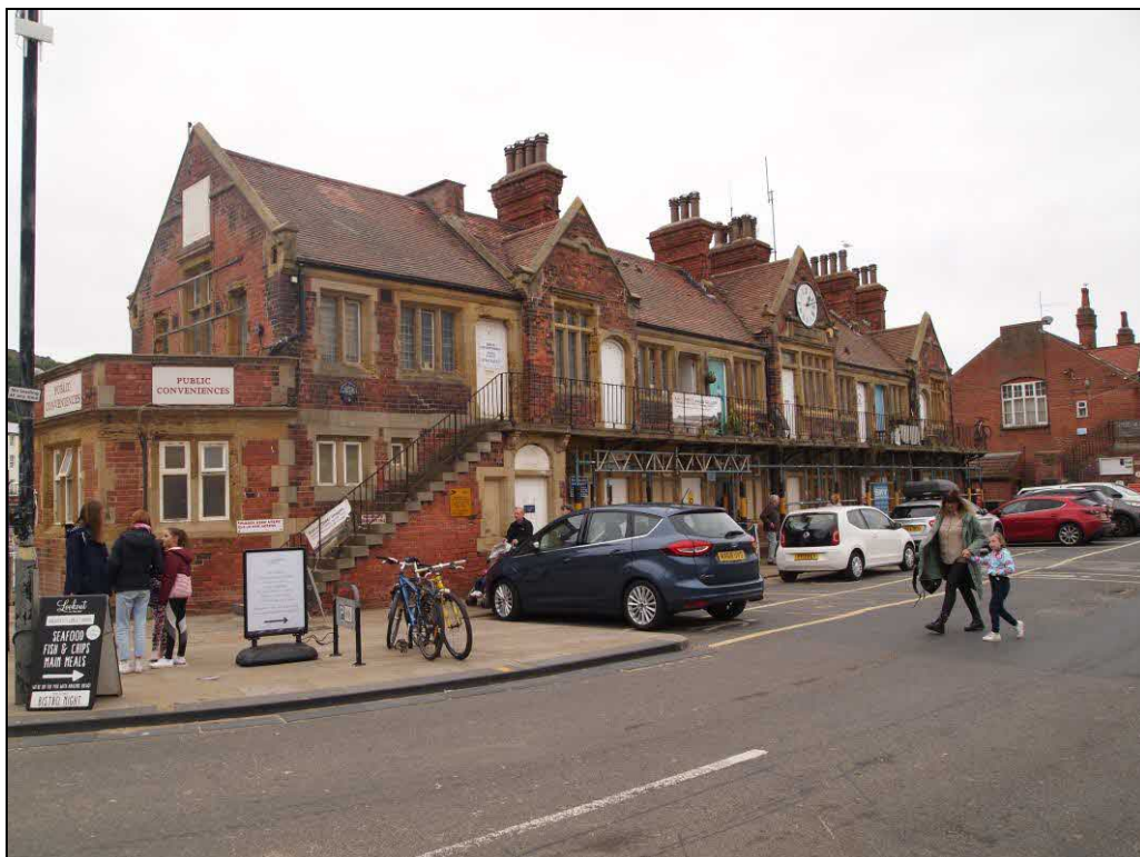
Figure 5: Building 1 front elevation.
