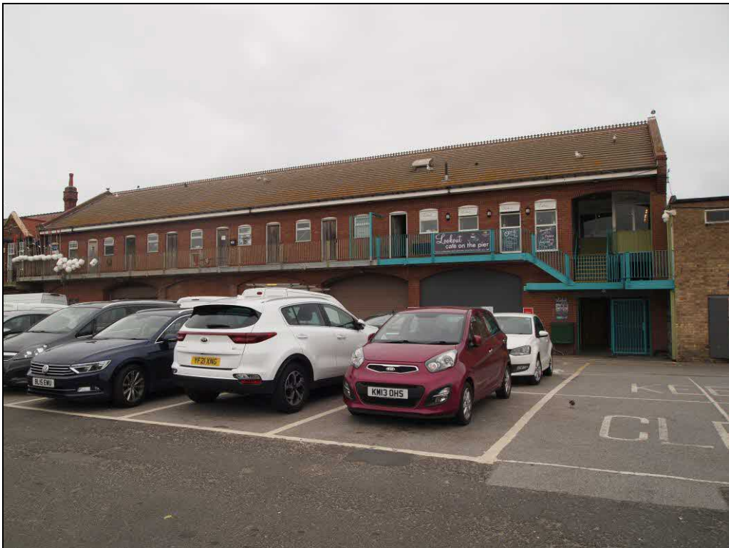
Figure 11: Building 3 front elevation.
