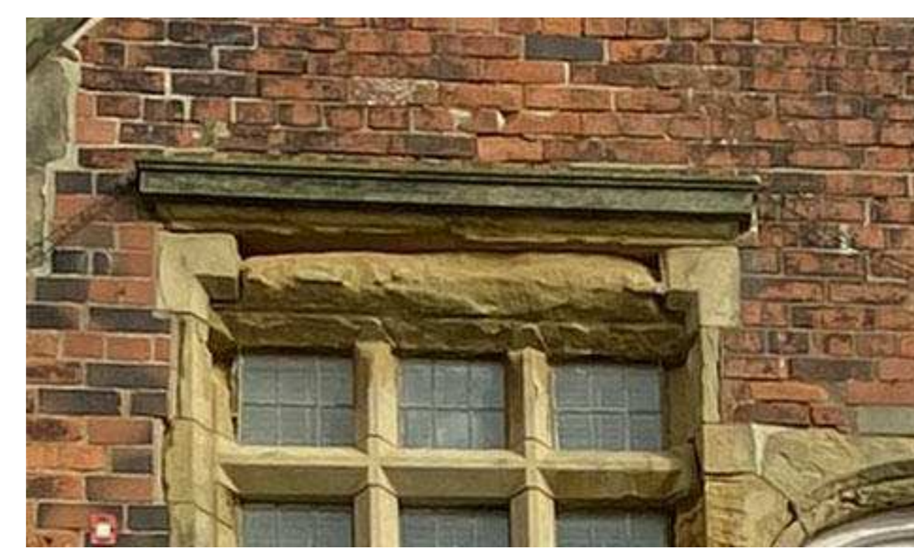
Example of stone window surround condition
