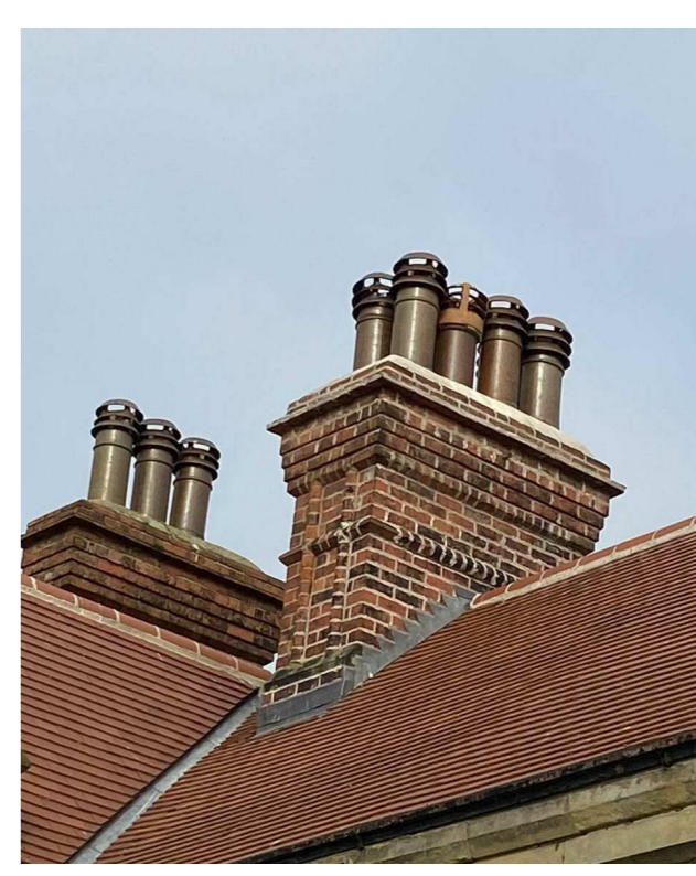
General condition of Chimneys
