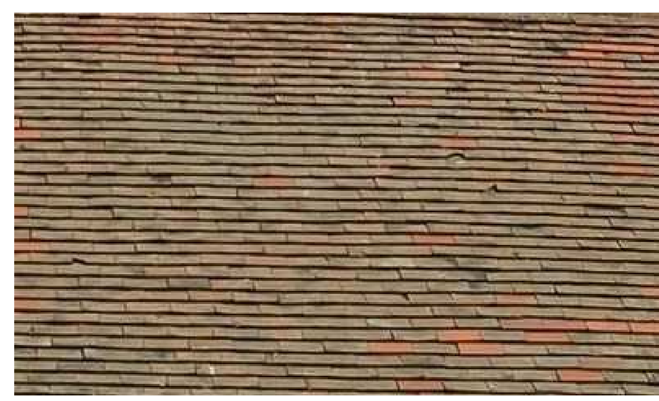
General condition of Roof Tiles
