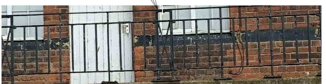
Example of Masonry to be cut-out and replaced
