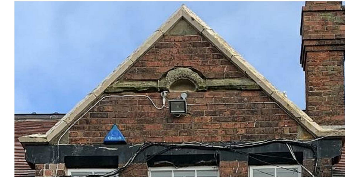
Condition of Gable Masonry
