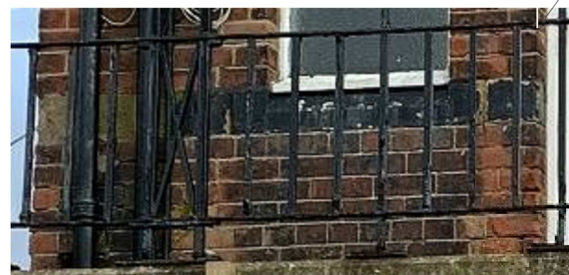
Example of Masonry to be cut-out and replaced
