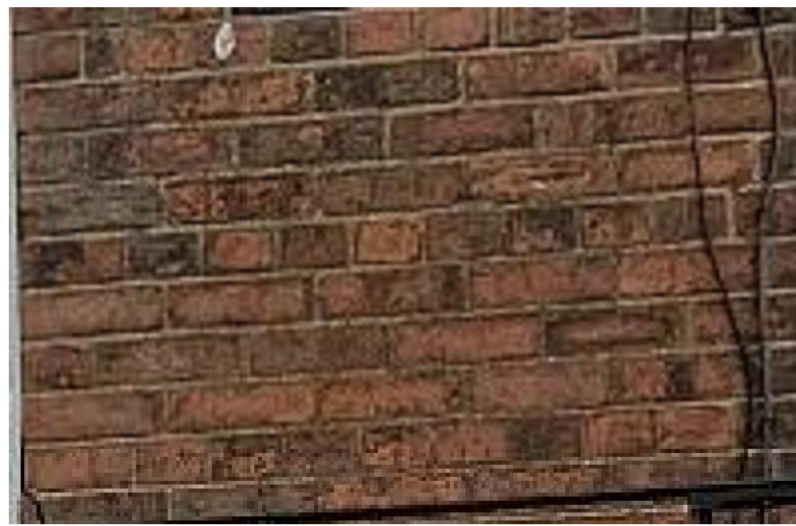
General condition of Brickwork to be cleaned
