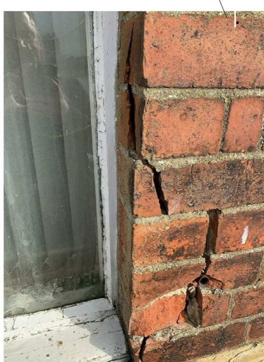
Example of Masonry to be cut-out and replaced
