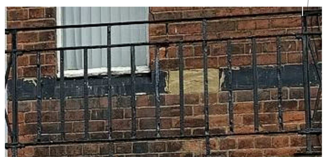
Example of Masonry to be cut-out and replaced
