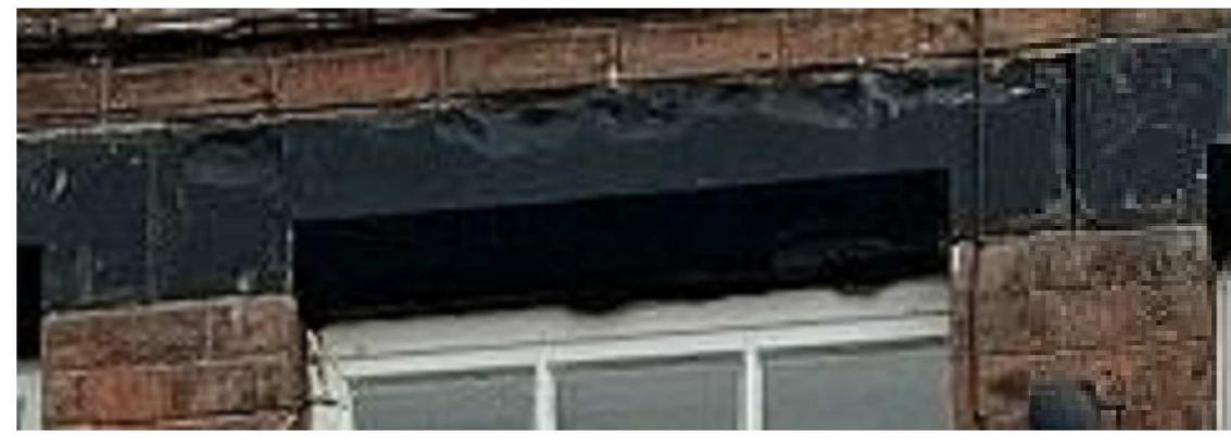
Condition of Stone Lintel to be replaced
