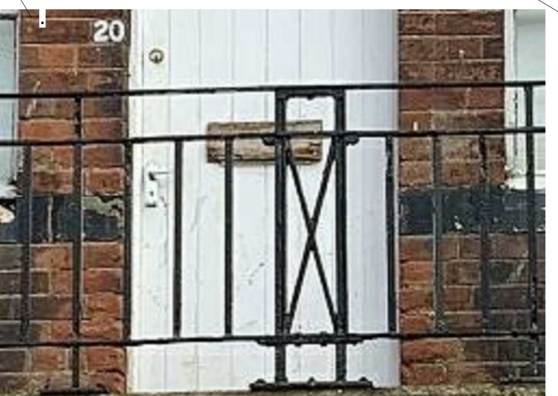
Example of Masonry to be cut-out and replaced
