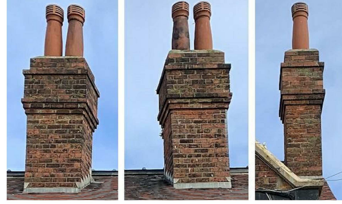
Condition of Chimneys
