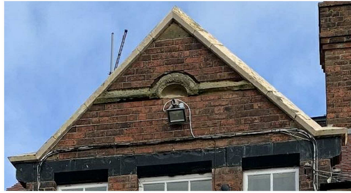
Condition of Gable Masonry
