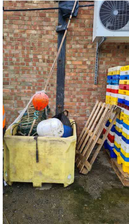
Figure General Image Showing the Storage of Materials/Equipment I Beam Severe corrosion / delamination
