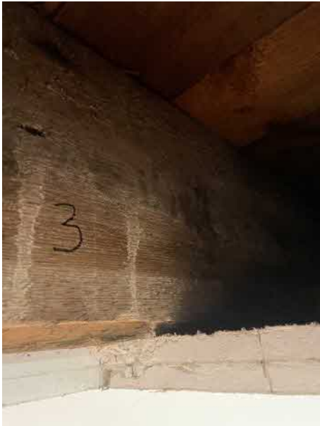
Figure Women's toilet location 3
