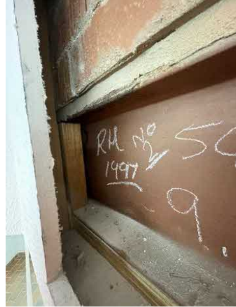
Figure Women's toilet location 2
