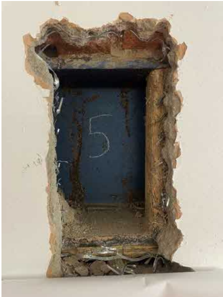
Figure Women's toilet location 5
