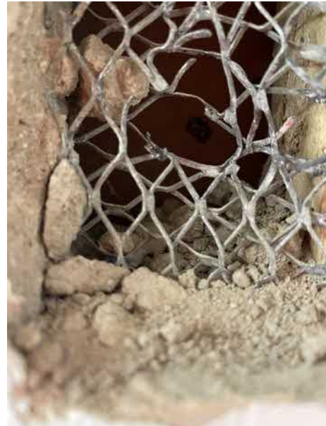
Figure Women's toilet location 7
