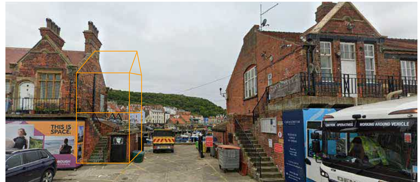
Building 1 from the West Pier Access Road
