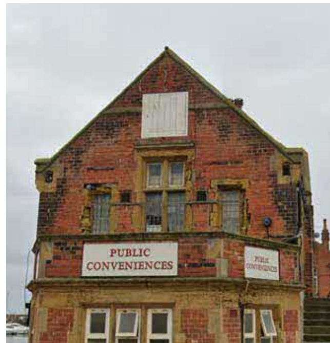
Building 1 North West Elevation 1st floor
