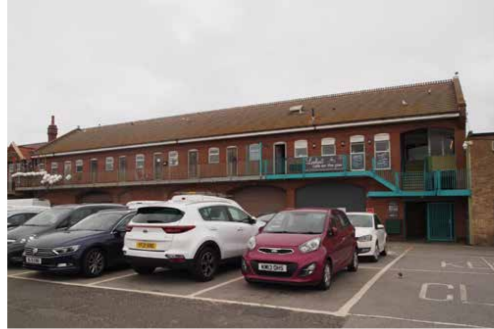
Building 3 (South-West facing)
