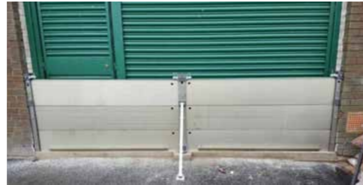
EXAMPLE DEMOUNTABLE ALUMINIUM FLOOD BARRIERS FOR DOORWAYS
