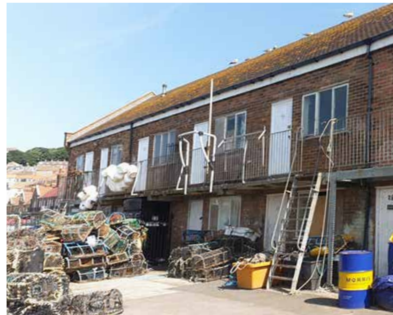
Bait Sheds - Building 5
