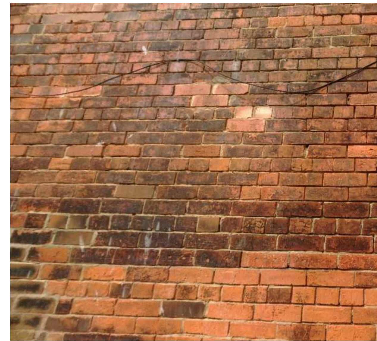
Example of General Masonry Condition
