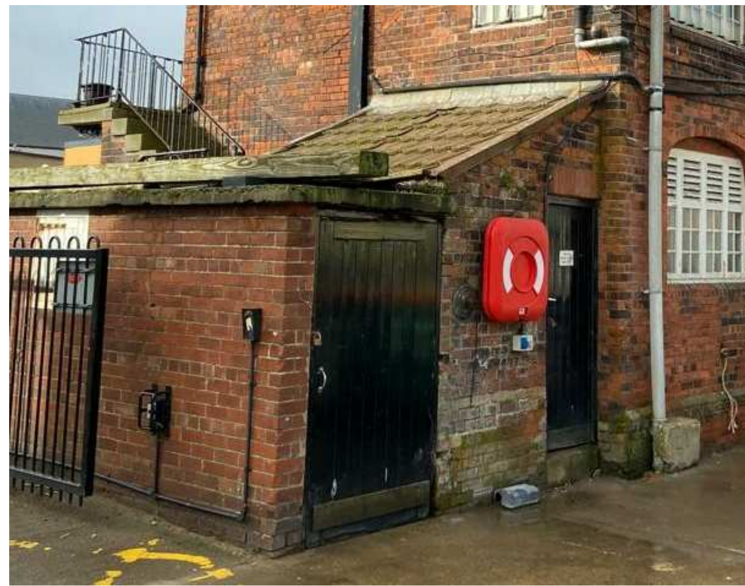
Outbuilding to be demolished as part of proposed works
