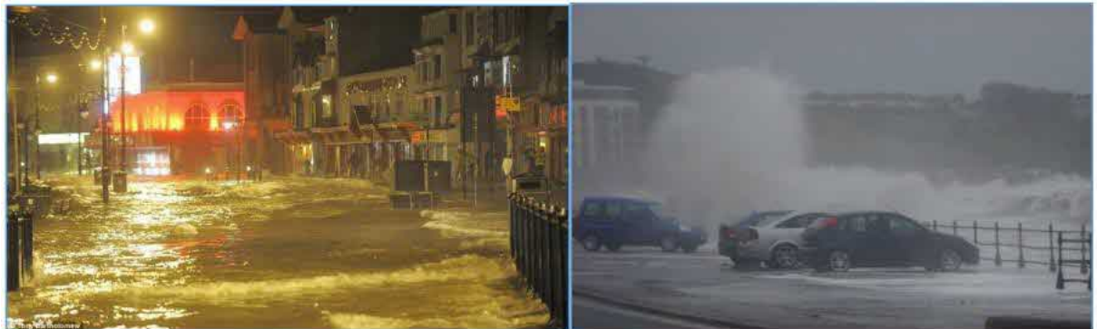
Figure 1-7: Scarborough seafront inundation 05/12/2013, (Left) and overtopping at Royal Albert Drive, 09/03/2009 (Right)
