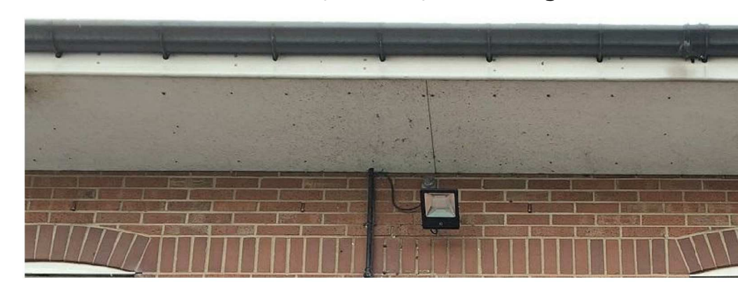
Common appearance / condition of Fascias, Soffits, Guttering
