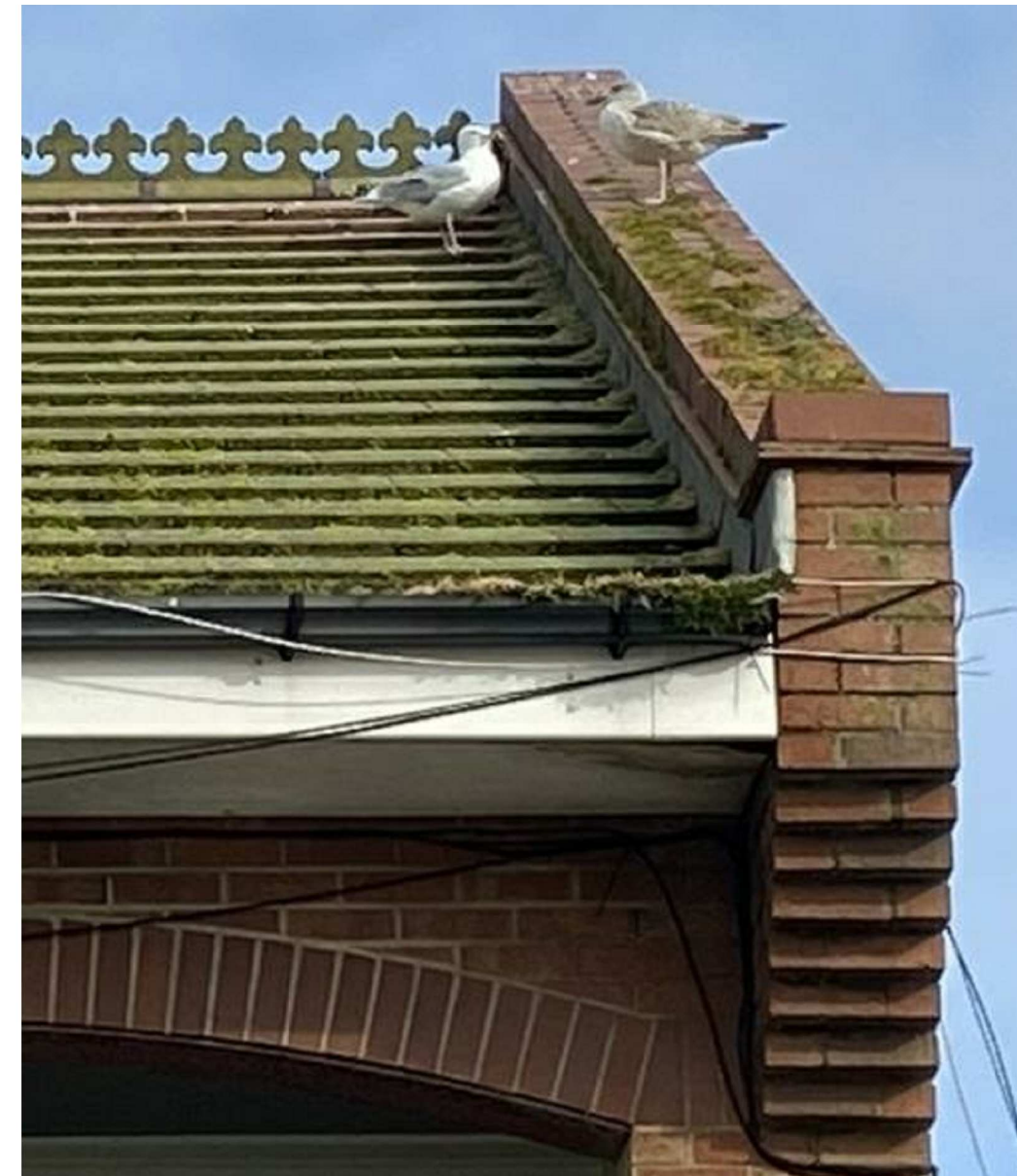
Common appearance / condition of Gable Copings
