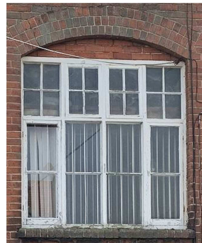
Windows to NW Elevation
