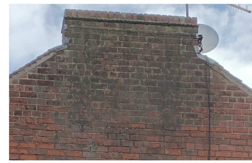
Example of level of brickwork cleaning required
