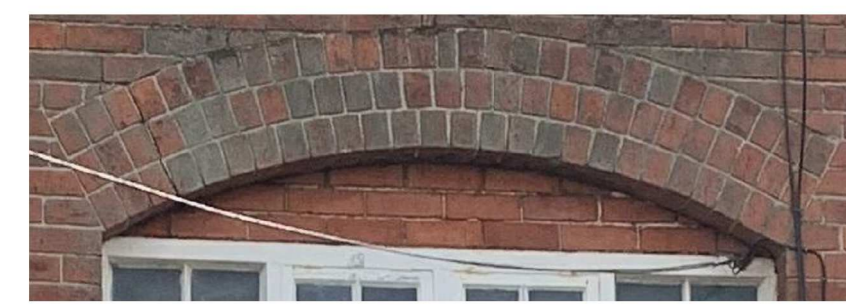
Brick infill to Window Head
