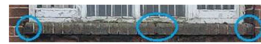
Brick Cill Repairs
