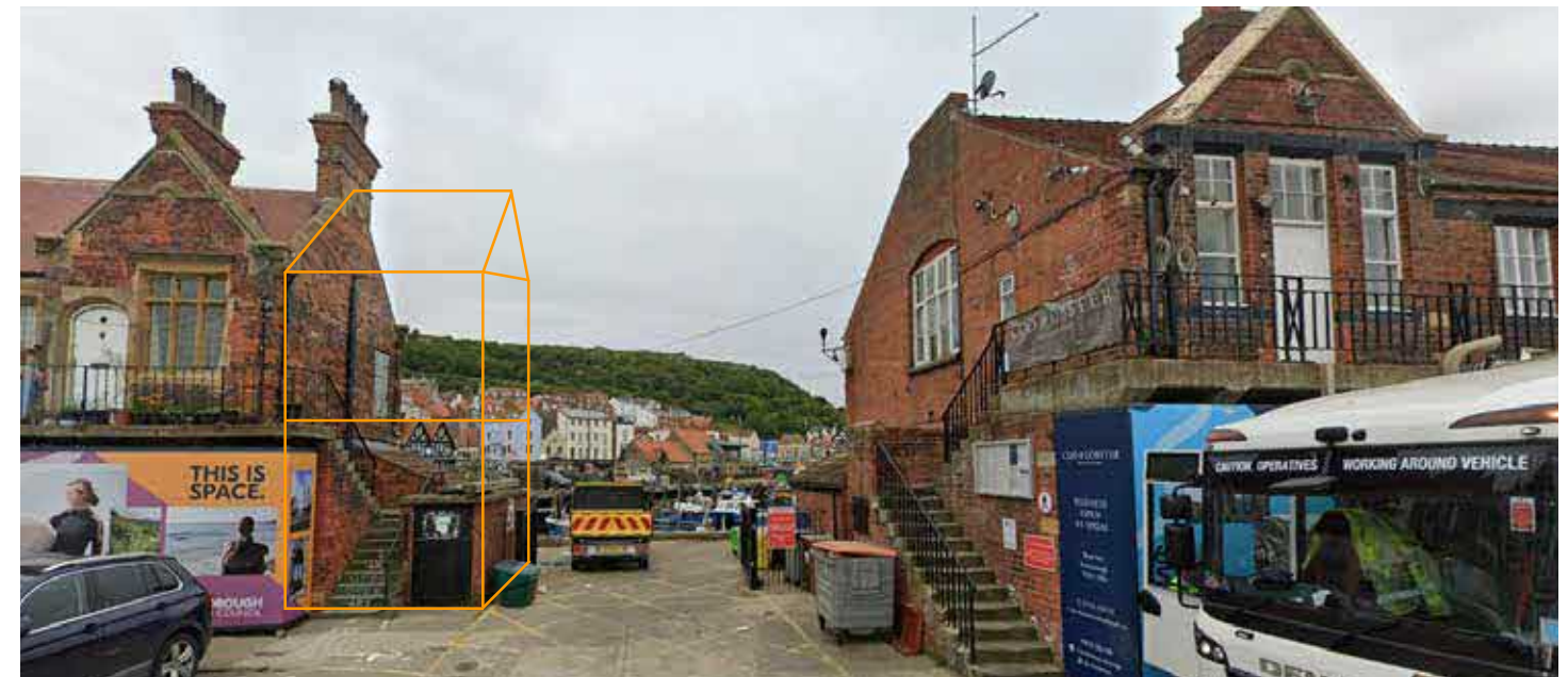
Building 1 from the West Pier Access Road
