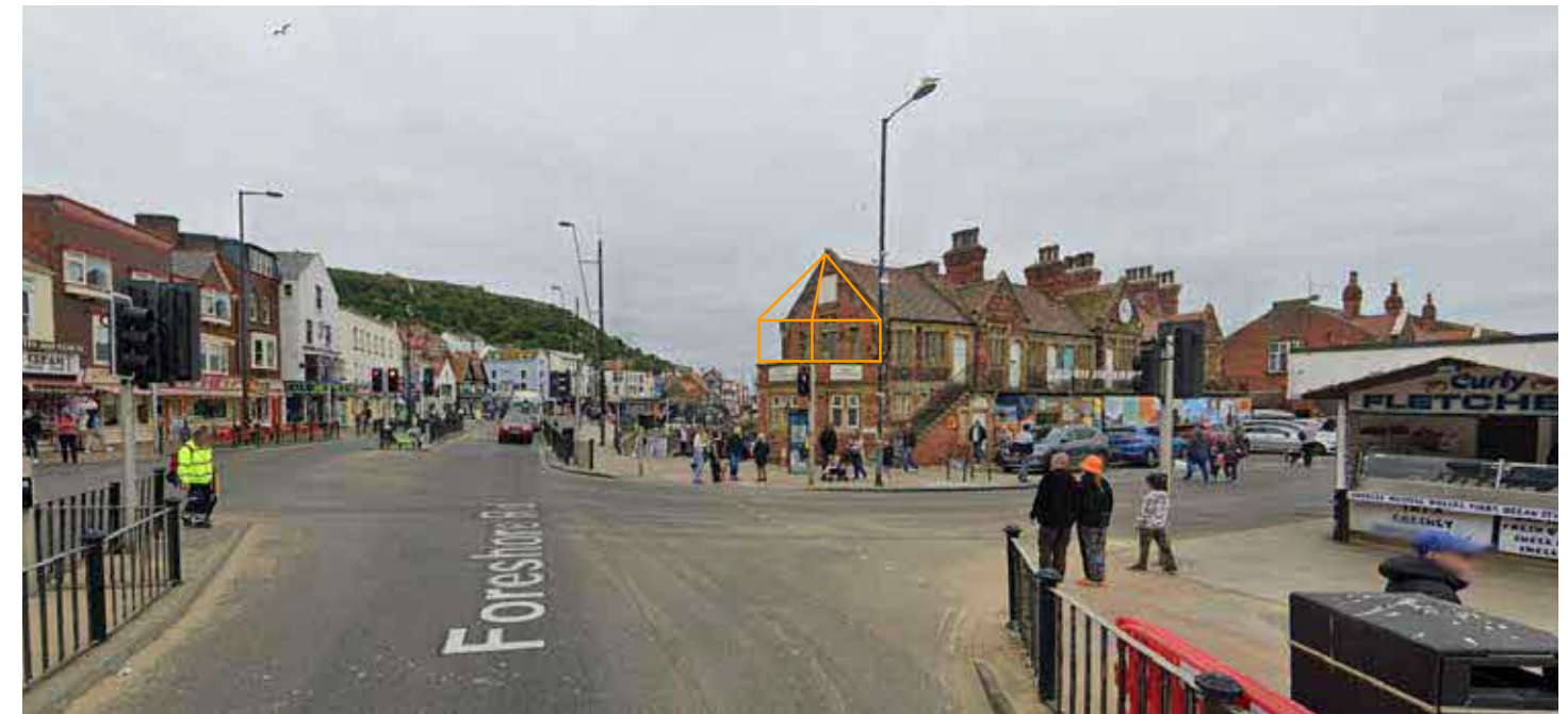
Building 1 from Foreshore Road
