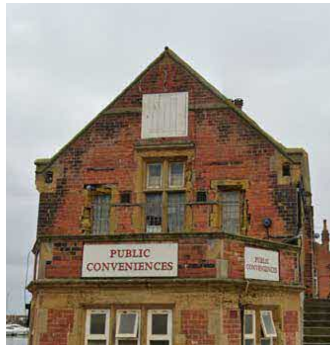
Building 1 North West Elevation 1st floor
