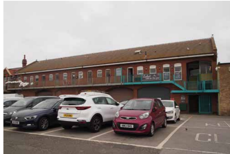
Building 3 (South-West facing)
