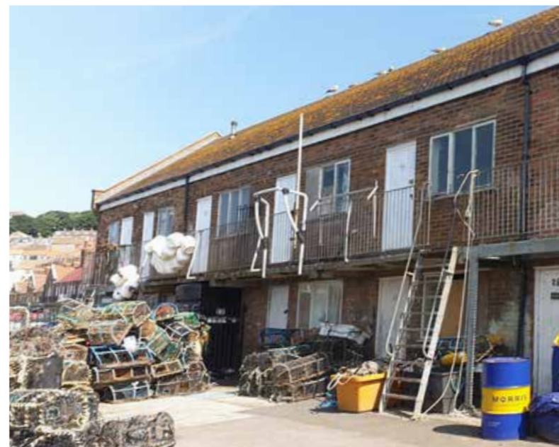
Bait Sheds - Building 5
