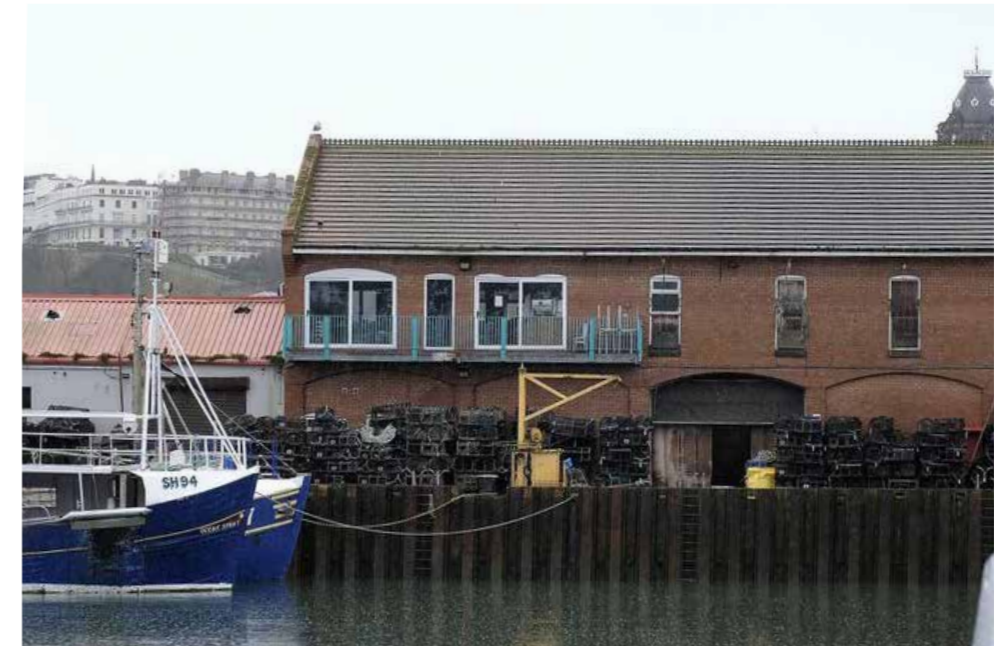
Lookout on the Pier - Building 3 (North-East facing)
