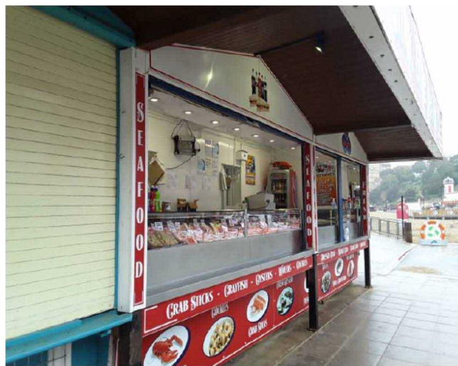
Photo 17 - North-west elevation showing overhang soffit and steel columns of Kiosks
