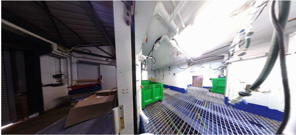
Photo 6 - Hygienic Wall Panels at ground floor Building 4a
