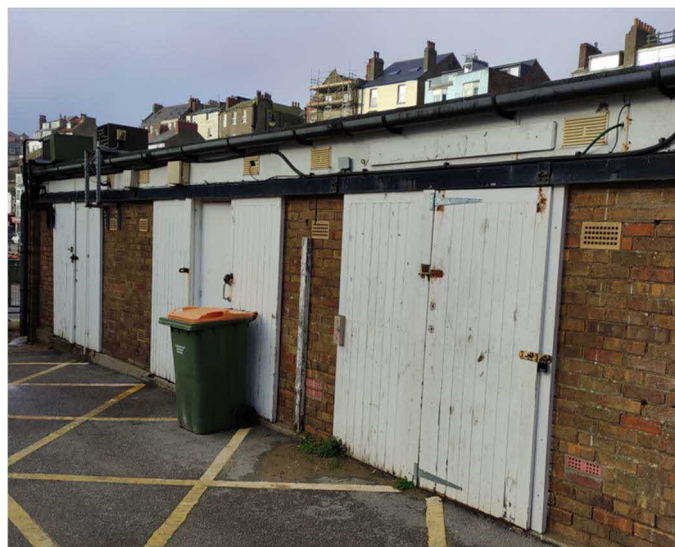
Photo 17 South-east elevation of Kiosks
