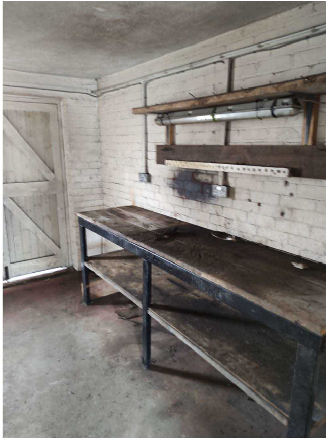
Photo 14 - Internal view of one unit at first floor level Building 7
