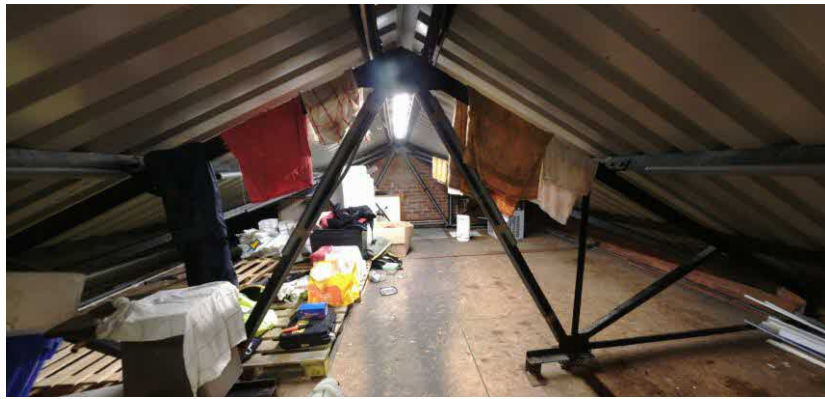
Figure 2 Building 4a Roof Truss
