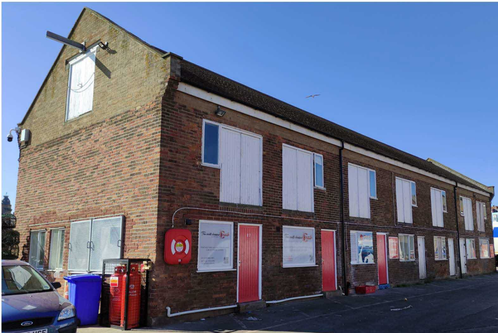
Photo 13 - South-east elevation of Building 7
