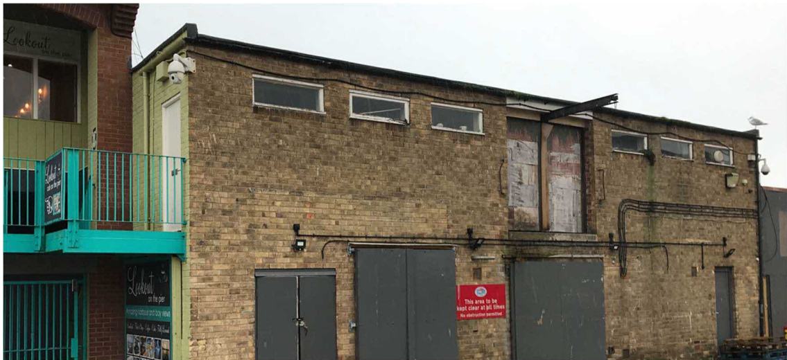
Photo 7 - South-west elevation of Building 4b
