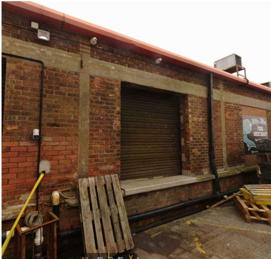
Photo 1 – South-west elevation of Building 4a
