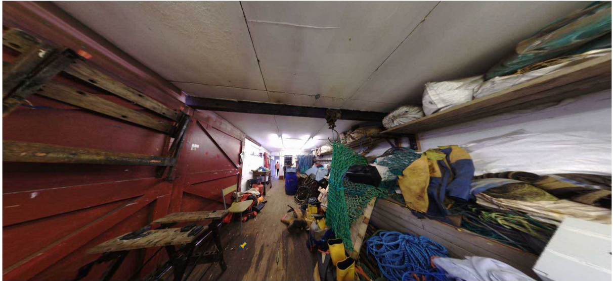
Photo 8 – Upper floor of Building 4b
