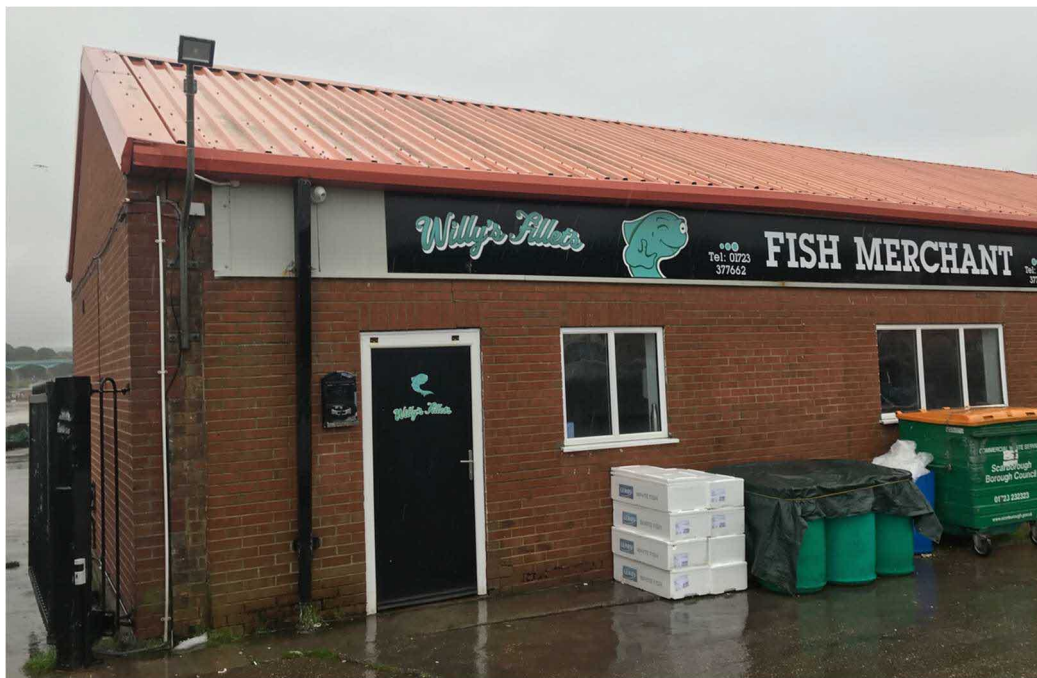
Photo 2 - North-east elevation of Building 4a
