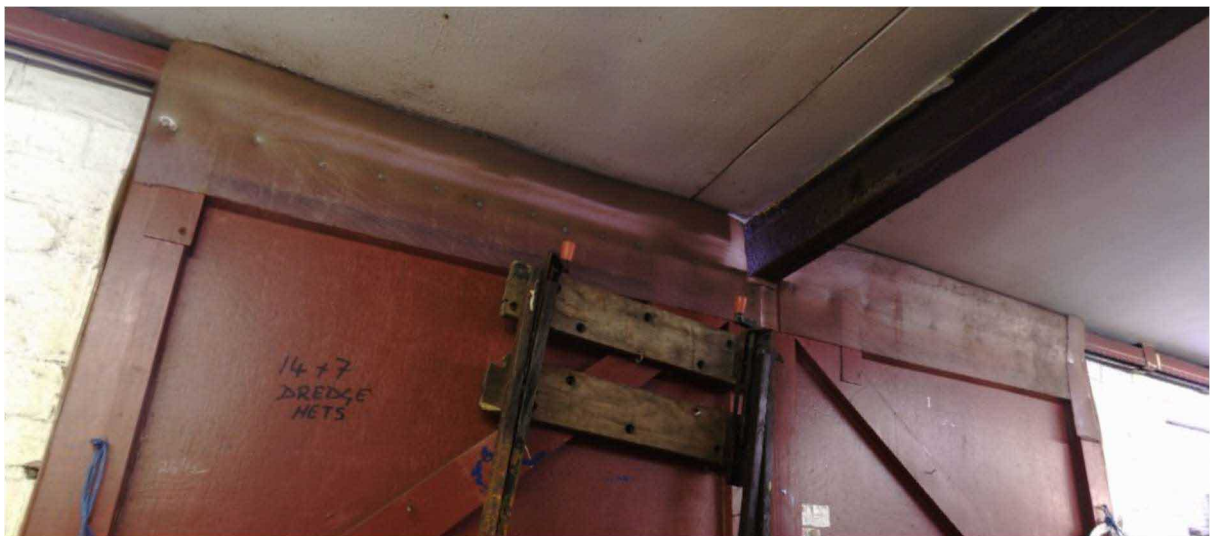
Photo 8 - Lifting Beam taken from inside Building 4b
